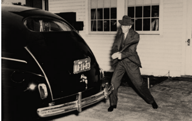
Figure 1.1: Photo of Henry Ford demonstrating the strength of his soy-based wood composite car body by taking an axe to it.
