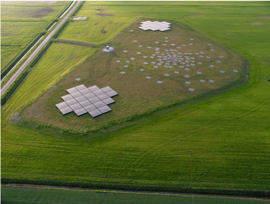
Figure 3–1: Dutch LOFAR substation. Note the two clusters of High Band Antennas in the foreground and background, and the quasi-randomly arranged Low Band Antennas in between. There are 24 High Band Antennas in Each cluster and 96 Low Band Antennas in the random dispersion [13].
