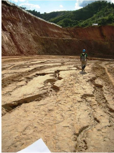
*Figure 1. Sheet erosion on the pipeline route in Ambatovy, in the vicinity of the mine, 2009*
