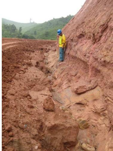
*Figure 4. Example of gully erosion process along the pipeline route of Ambatovy, 2010.*
