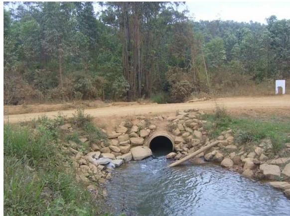
*Figure 10. Stream crossing using a culvert*
