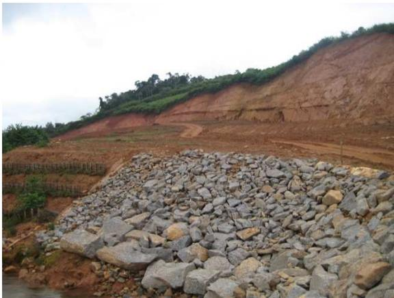
*Figure 9. Bank stabilization*
