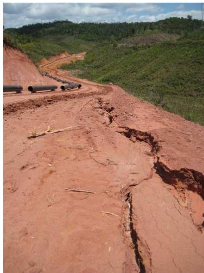
*Figure 2. Example of interrill erosion process along the pipeline route of Ambatovy.*
