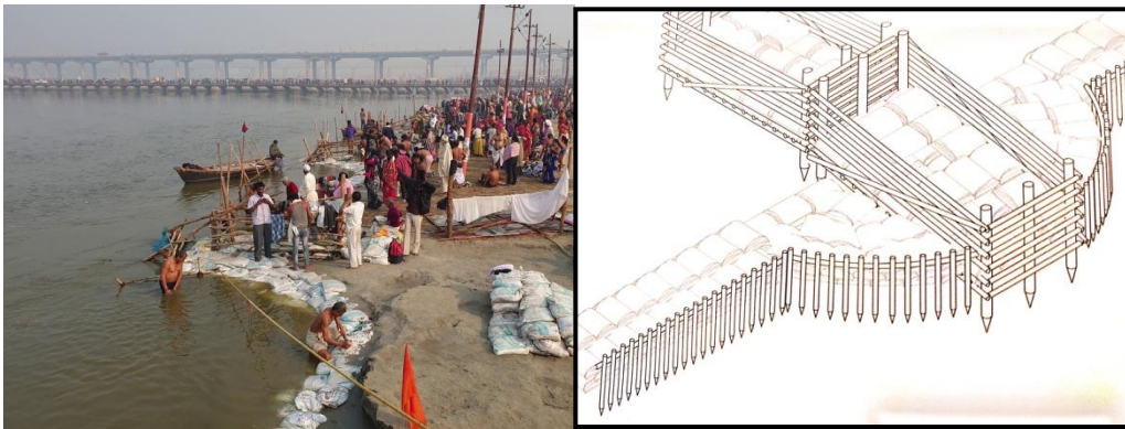
Fig. 83 (left): The beginning of the process by lining the sandbags to form the edge (R. Mehrotra & Vera, 2015).
