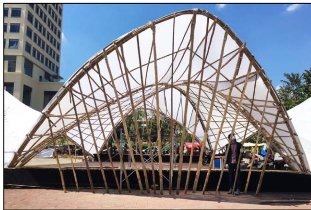
Fig. 29: A hyperbolic pavilion where the bamboo's ductility allows the structure to bend and the fabric's foldability, lightness and tensile character allows it to act as a roof of the structure Photo: Building
