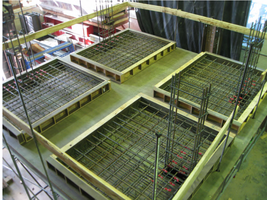
Figure 3.17: Assemblage of reinforcement before first concrete placement
