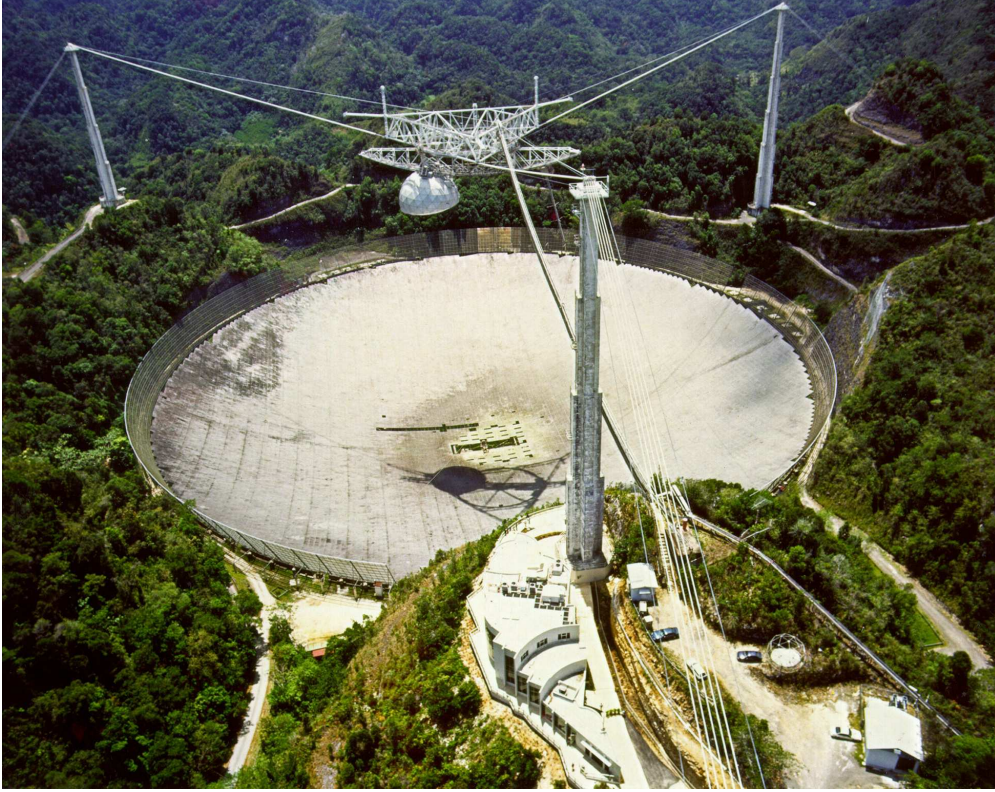
Figure 2.2: Arecibo Observatory William E. Gordon 305-m Telescope. One can see the steerable Gregorian dome suspended above the primary dish, which has a secondary and a tertiary reflector that focus the light into a single point, at the location of the ALFA instrument.
