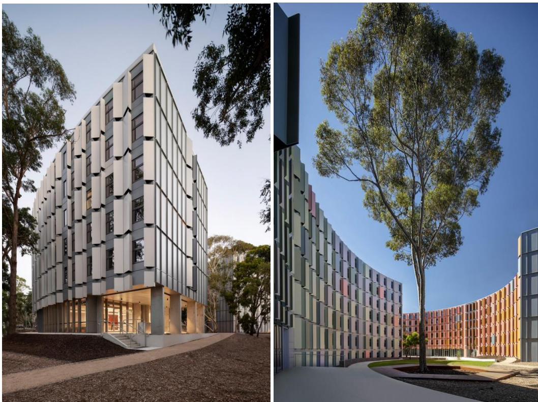
Figure 3.99: Prefabricated aluminum sun panels
