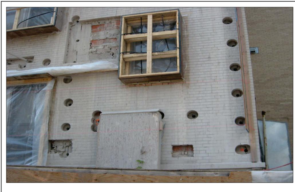
**Figure 25 - Close-up view of anchor locations before casting the shear wall**
