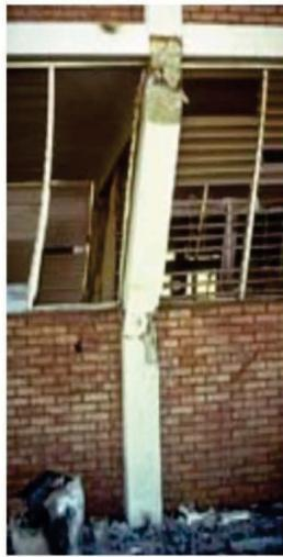
**J84.** Two-story reinforced concrete building, Managua, Nicaragua, damaged in the 1972 Managua Earthquake. The slide shows a reinforced concrete column which was part of the structural system and which failed due to its shortening because of the effect of the masonry wall. The masonry walls were considered as non-structural elements.
