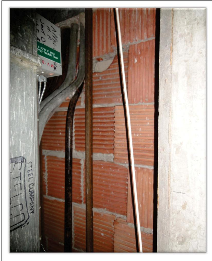
**Figure 1 - Terra Cotta infill masonry wall in CHU Sainte-Justine in Montréal (Asgarian, 2010)**
