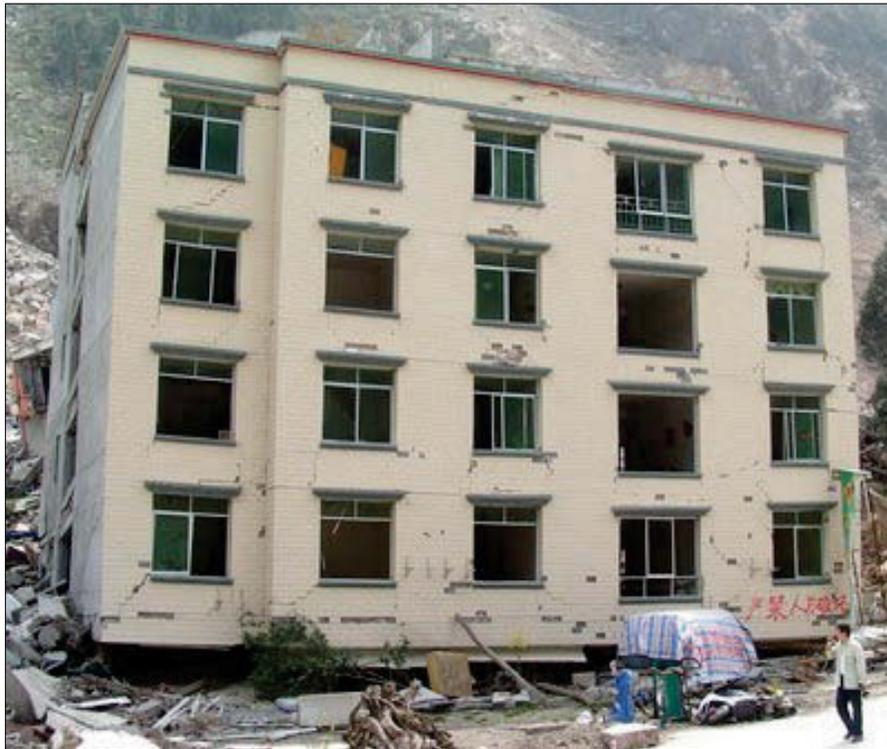
**Figure 3 - Failure due to creating the soft first storey, Beichuan, China, 12 May 2008 earthquake [42]**
