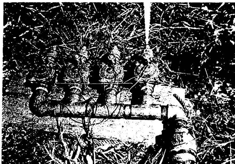
Figure 2a Electric Valve Manifold for Simulation of Field Lateral Discharge When Recycling Irrigation Water to Offset Pond
