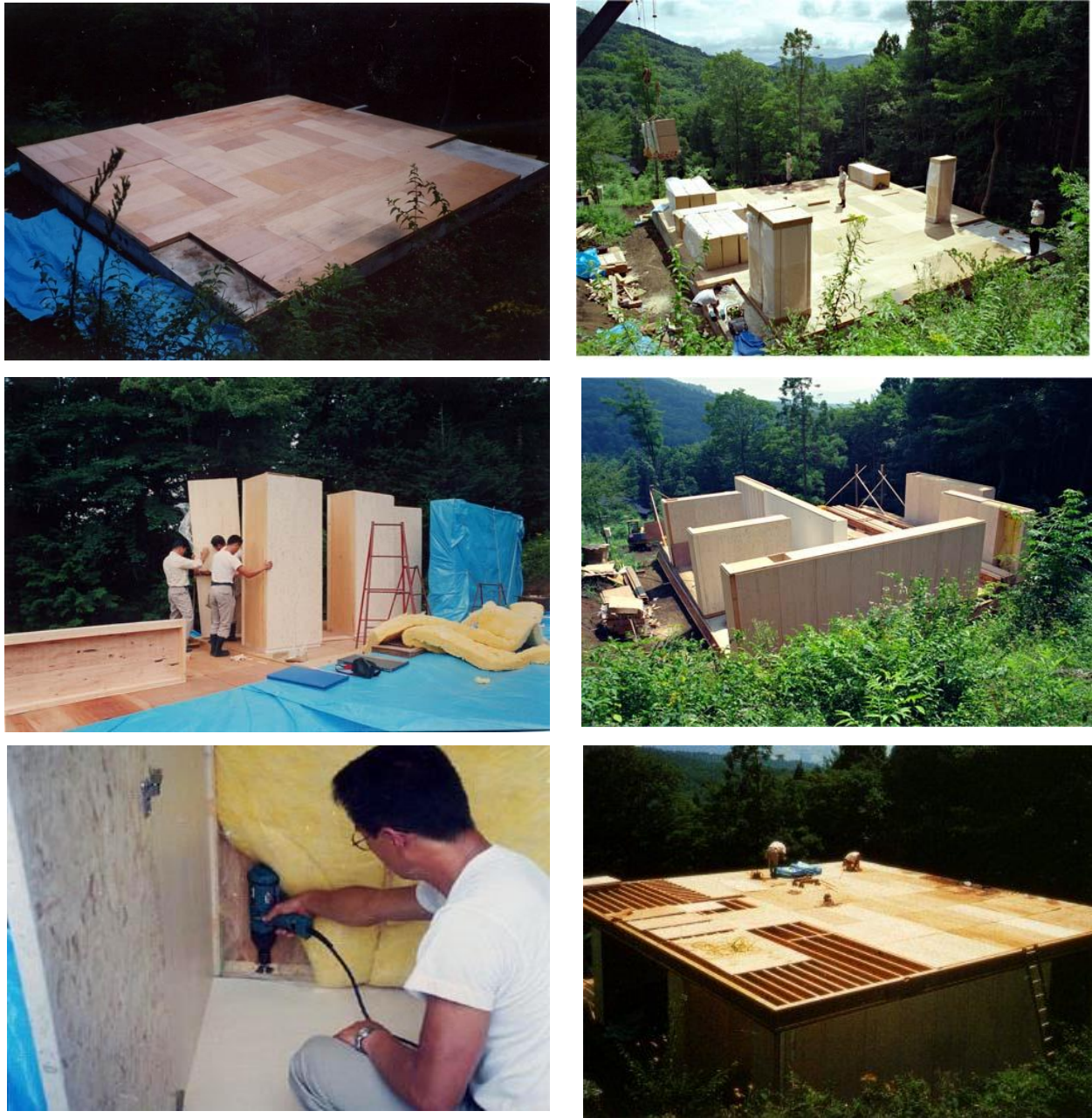
Figure 3.53: Construction process of the Furniture House 1. Source: Shigeru Ban Architects, http://www.shigerubanarchitects.com/works/1995_furniture-house-1/index.html
