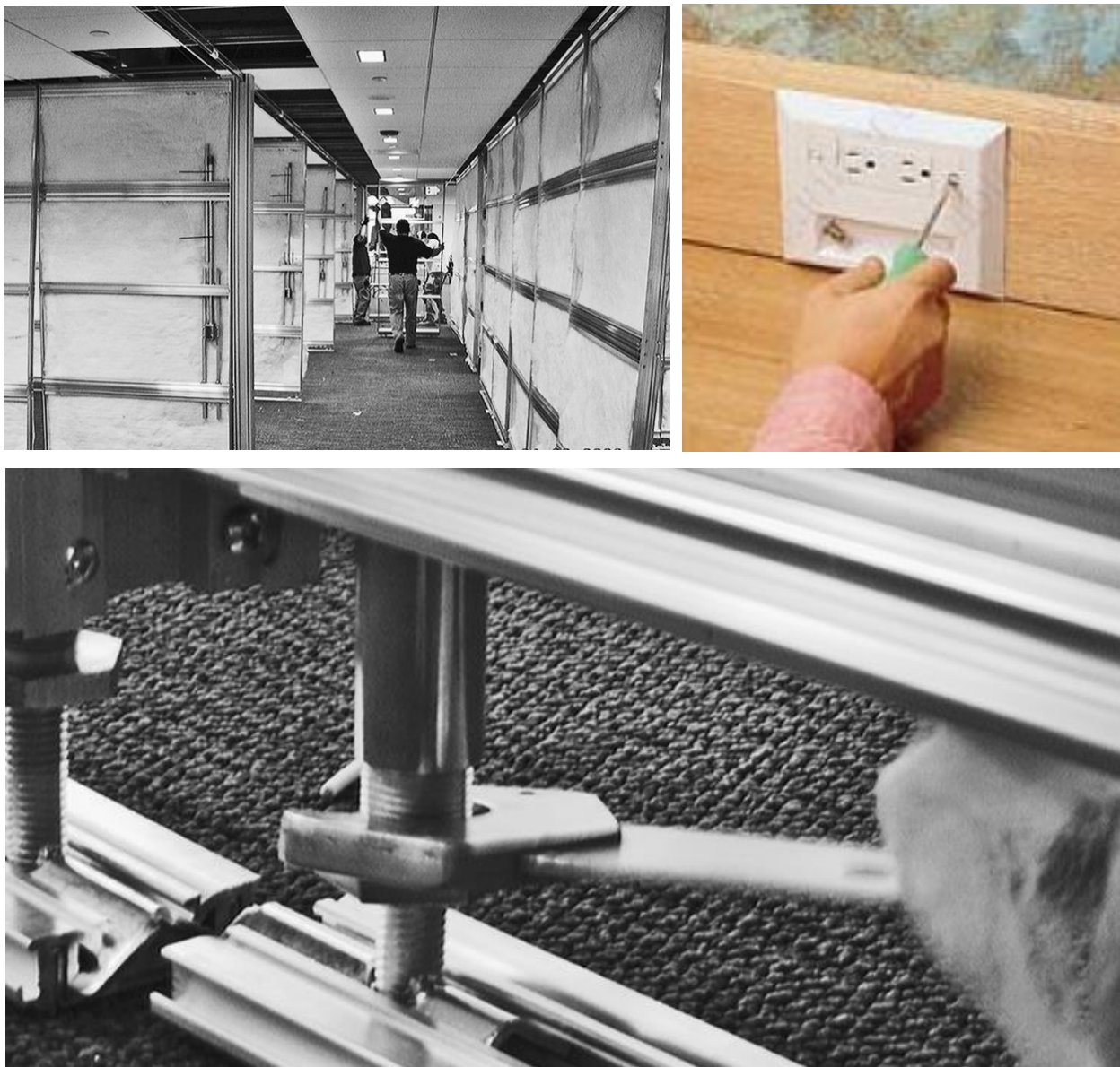
Figure 2.9: Top Left: DIRT TM interior partition system; Top Right: Cable Raceway; Bottom: DIRT TM Floor mounted panels, Sources: Smith, 2010, pp.158.
