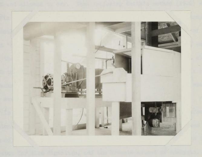
Fig. 2. Laboratory sprayer seen through screened wall of insectary Left, motor, pump, and spray tank. Right, spindle chamber showing motor and gear box beneath. Tip of spray nozzle and lever operating quick-opening valve show directly behind plate attached to end of chamber.
