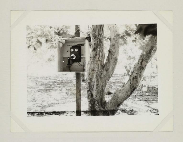
Fig. 17 Field telephone, one of several used to facilitate communication between spray shed and spray gun operators.
