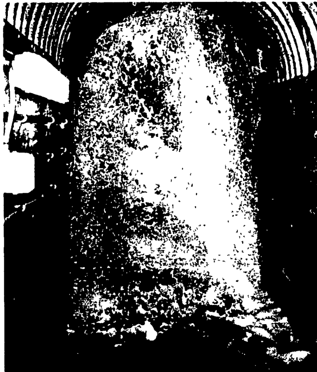
FIGURE 8.12 - WATER LEAKING INTO FOUNDATION GALLERY AT FULL RESERVOIR, STATION 25+20
