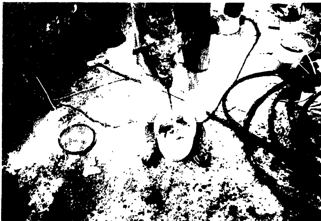
FIGURE 8.35 MIXING THE EPOXY PASTE WITH A DRILL MOTOR PADDLE MIXER
