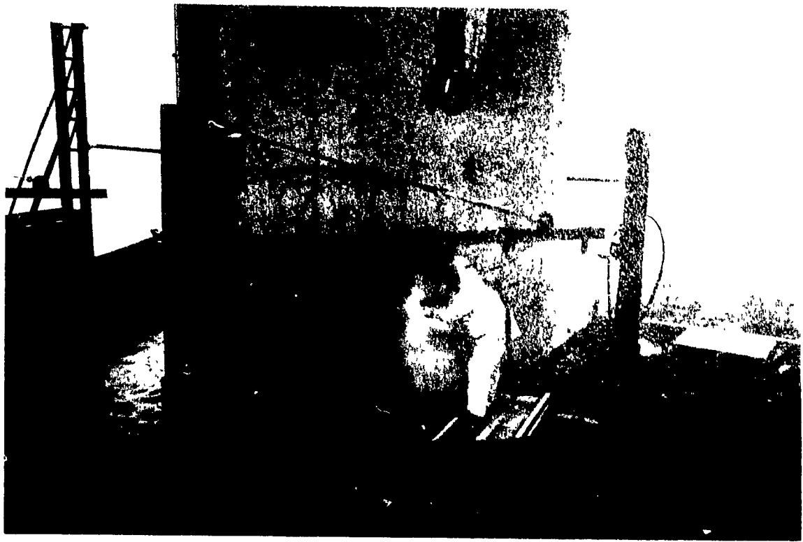
FIGURE 8.33 - CLEANING CRACKS WITH A HIGH PRESSURE WATER JET
