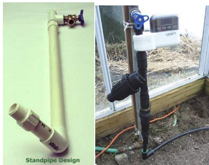
Standpipe installed with timer and filter
