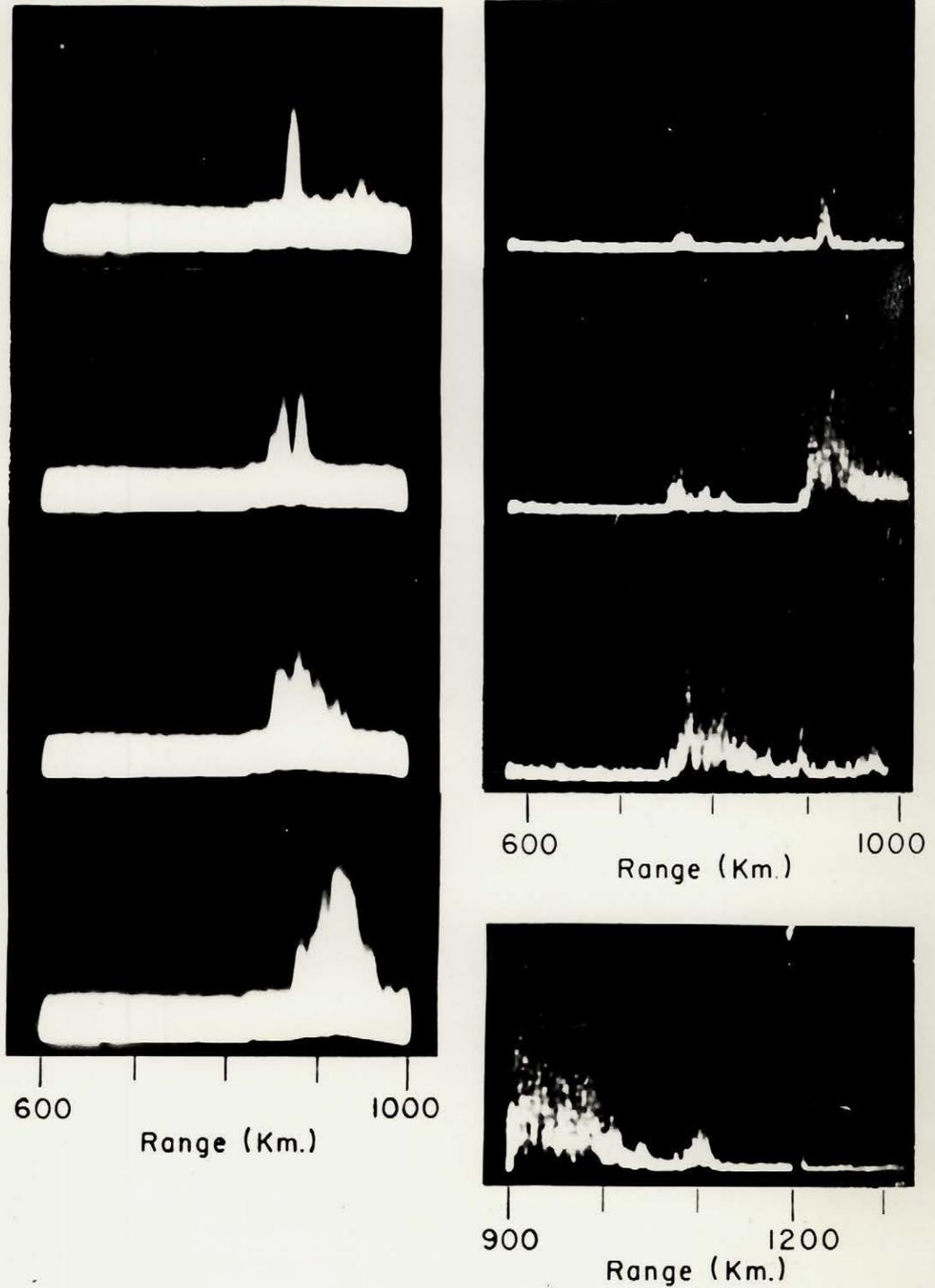
Figure 4.01 - Typical photographs of the range display showing auroral echoes. Those in the left hand column were taken with long exposures to show the outline of the echo, whereas the others were taken with short exposures to show the fine structure.
