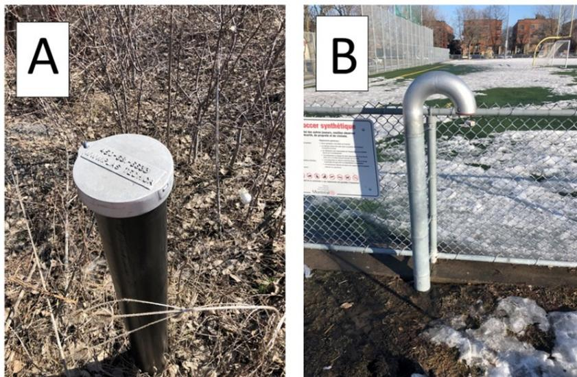
**Figure 5.7:** Photos of two CH<sub>4</sub> source types encountered at some historic landfill locations: A) observation well with locked cap; B) J-shaped metal vent surrounding an Astroturf outdoor recreation facility built over a historic landfill site.
