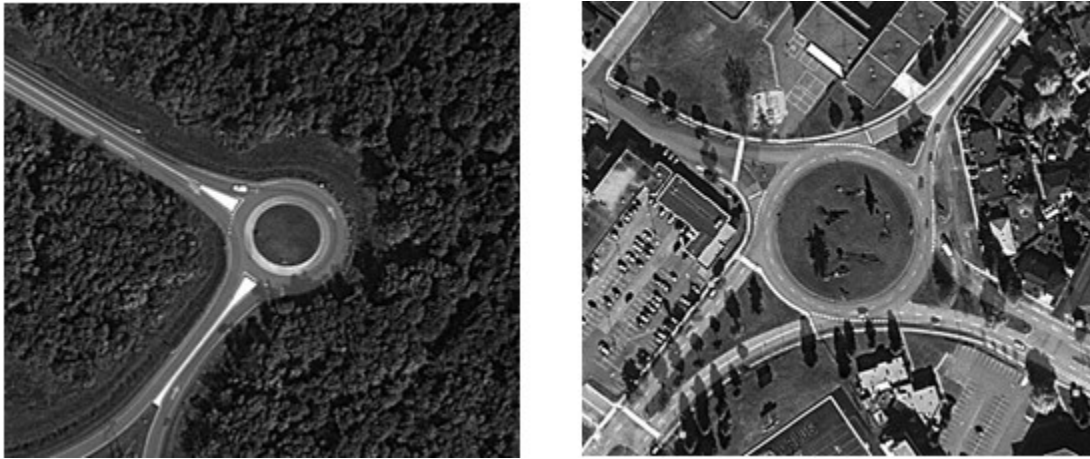
FIGURE 3: Roundabout-type intersections; Bromont, QC (left) and Trois-Rivières, QC (right) (15).
