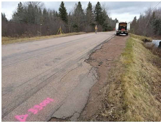
Figure 24. The effect of storm waters and soil erosion after large storm even in Haute-Aboujagane 112
