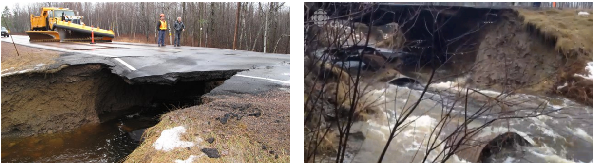
Figure 22. Storm water washes out sections of roads in southeast New Brunswick 108
