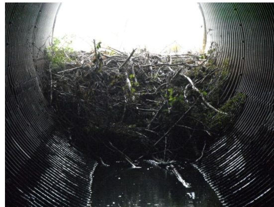
Figure 25. Beaver dam blocking culvert A060 113
