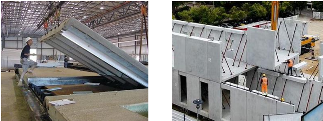
Figure 1-1 Precast Concrete Systems: Factory Fabrication and On-Site Assembly
