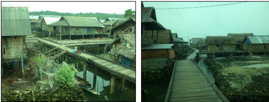
Figure 4.3: Photos of the government-funded bridge in Sama Bahari. Source: Author.
