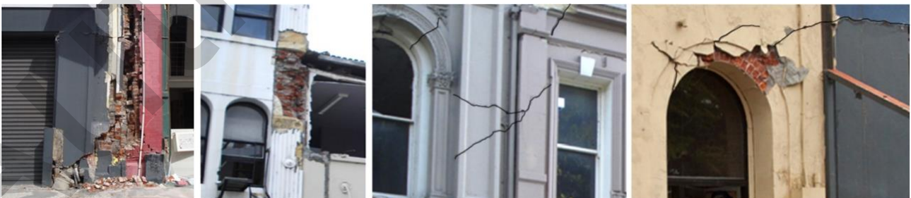
37 Figure 1. Pounding damage in URM buildings after the 2011 Christchurch earthquake (Cole et al. 2010)
