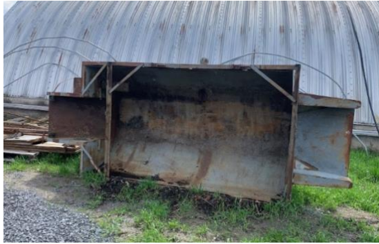
Figure 10. Initial Steel Structure
