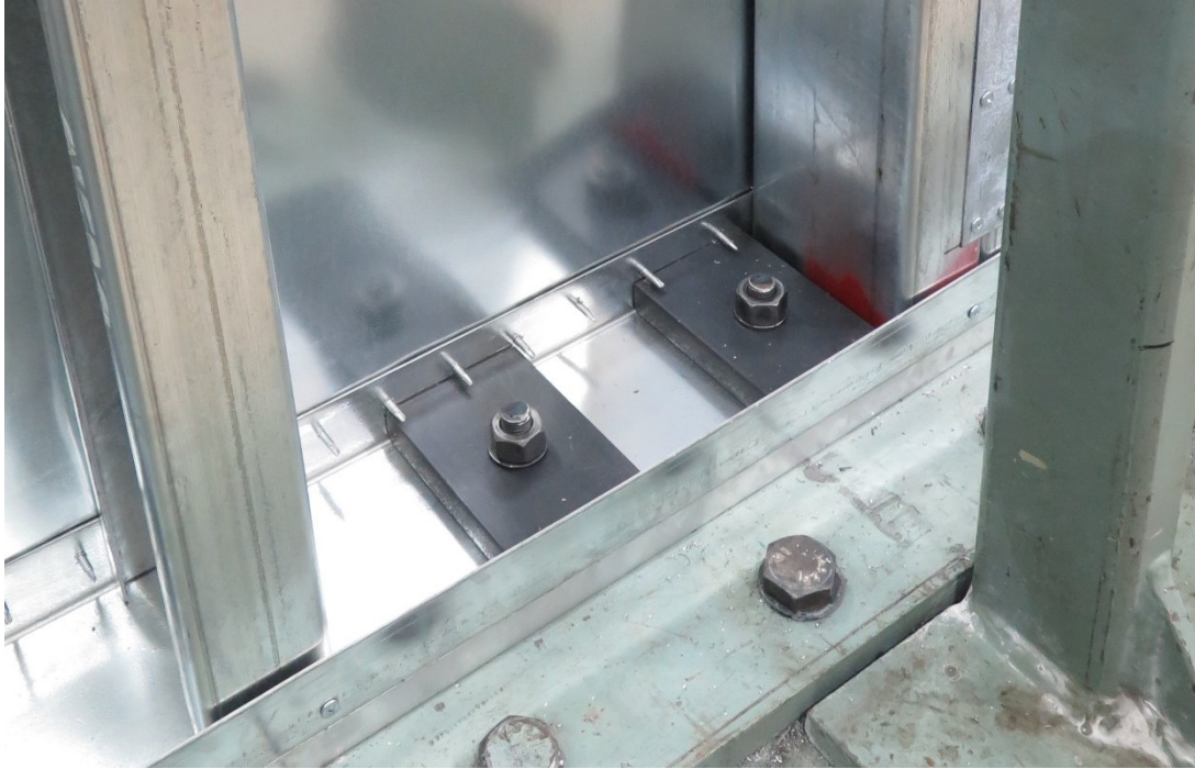
Figure B-5 Double-sheathed configuration: steel plates at shear anchors position (photo taken prior to installation of second sheathing member)
