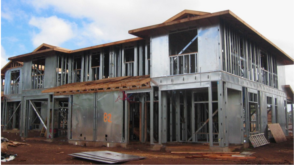
Figure 1.1 Cold-formed steel used as structural members and cladding for a house using CFS shear walls as SFRS (photo courtesy of J. Ellis, Simpson Strong-Tie Co. Inc.)
