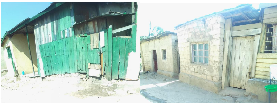
Figure 12. Old (left) timber and improved (right) cement block housing construction in Bannyahe
