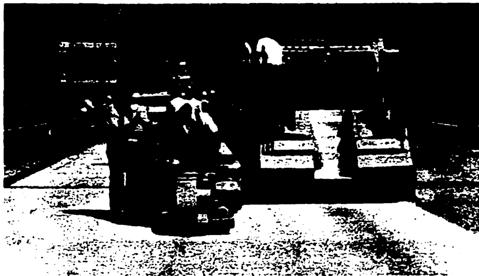
Figure 2.1 Shotblast equipment used to clean a deck [Sprinkel 1993]
