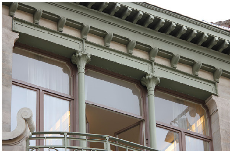
Fig. 1.21 - Hôtel Tassel, façade, detail of the two iron columns of the last storey [author's photograph, 2012]
