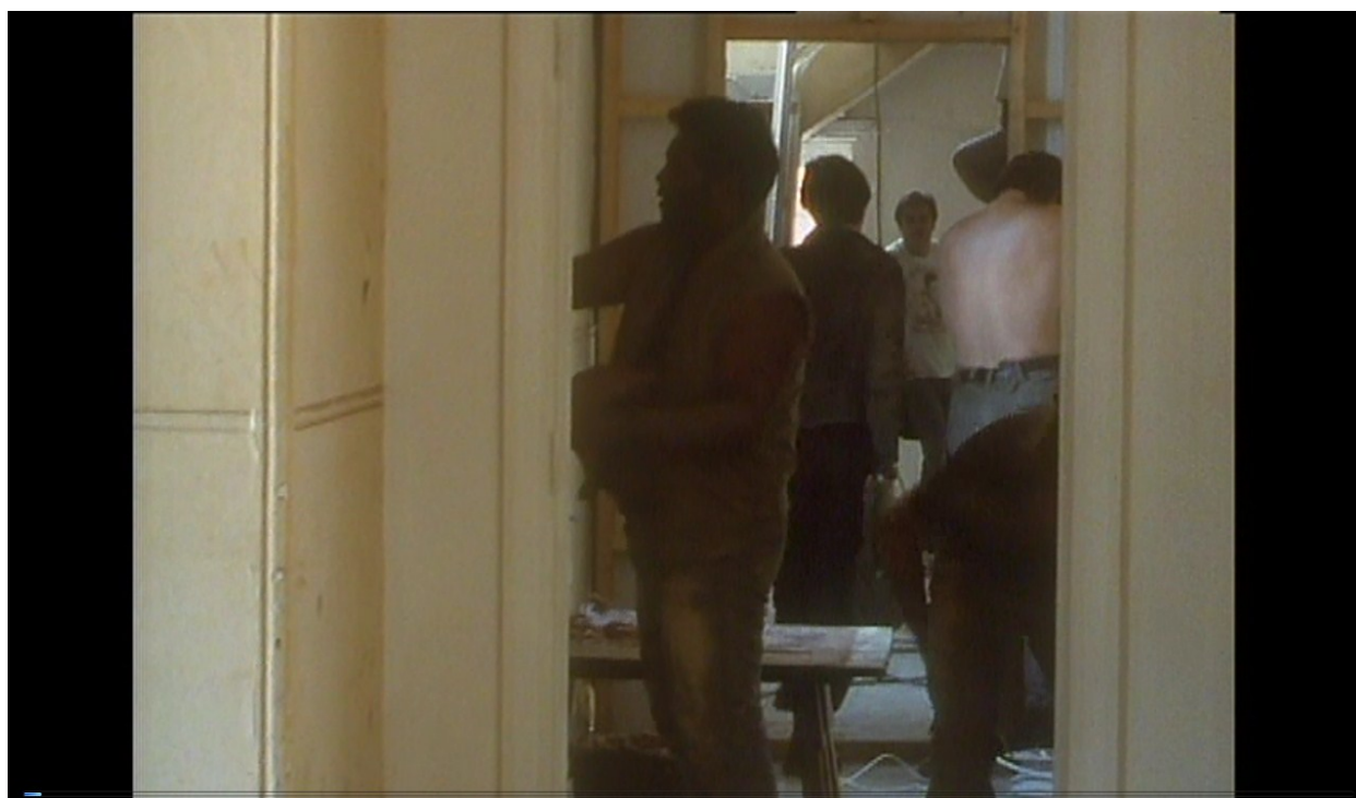
Interior shot showing the everyday tasks and working conditions on the building site
