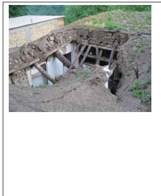
Fig. 2.27. The roof of a house: the point where destruction of the house usually begins. Photograph by author, 2008.
