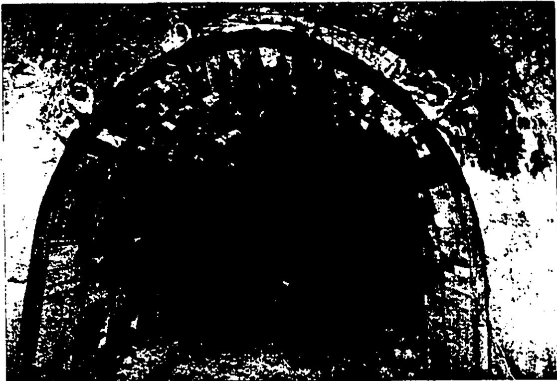
**Figure 4.4.4: Hollybank two-piece steel arches for drift support.**
