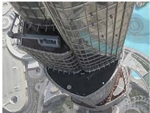
Figure 31: Outrigger walls in mechanical floor
