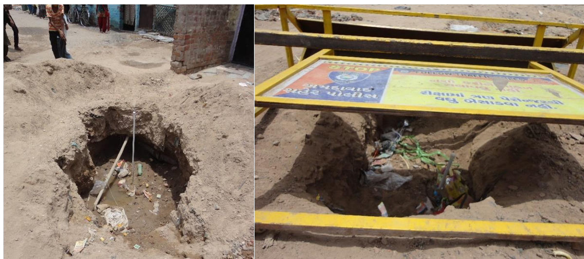
Figure 1. Abandoned and uncovered water pipe repairs in Ahmedabad
