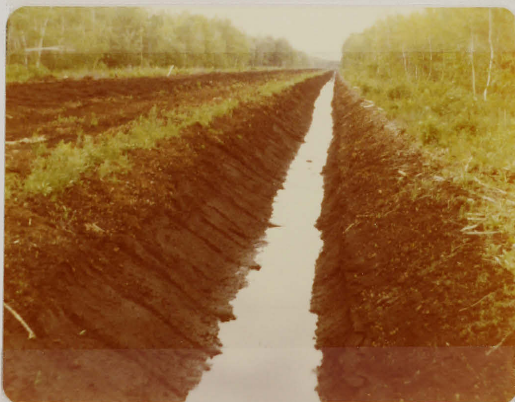
PHOTO 8. New drainage ditch
