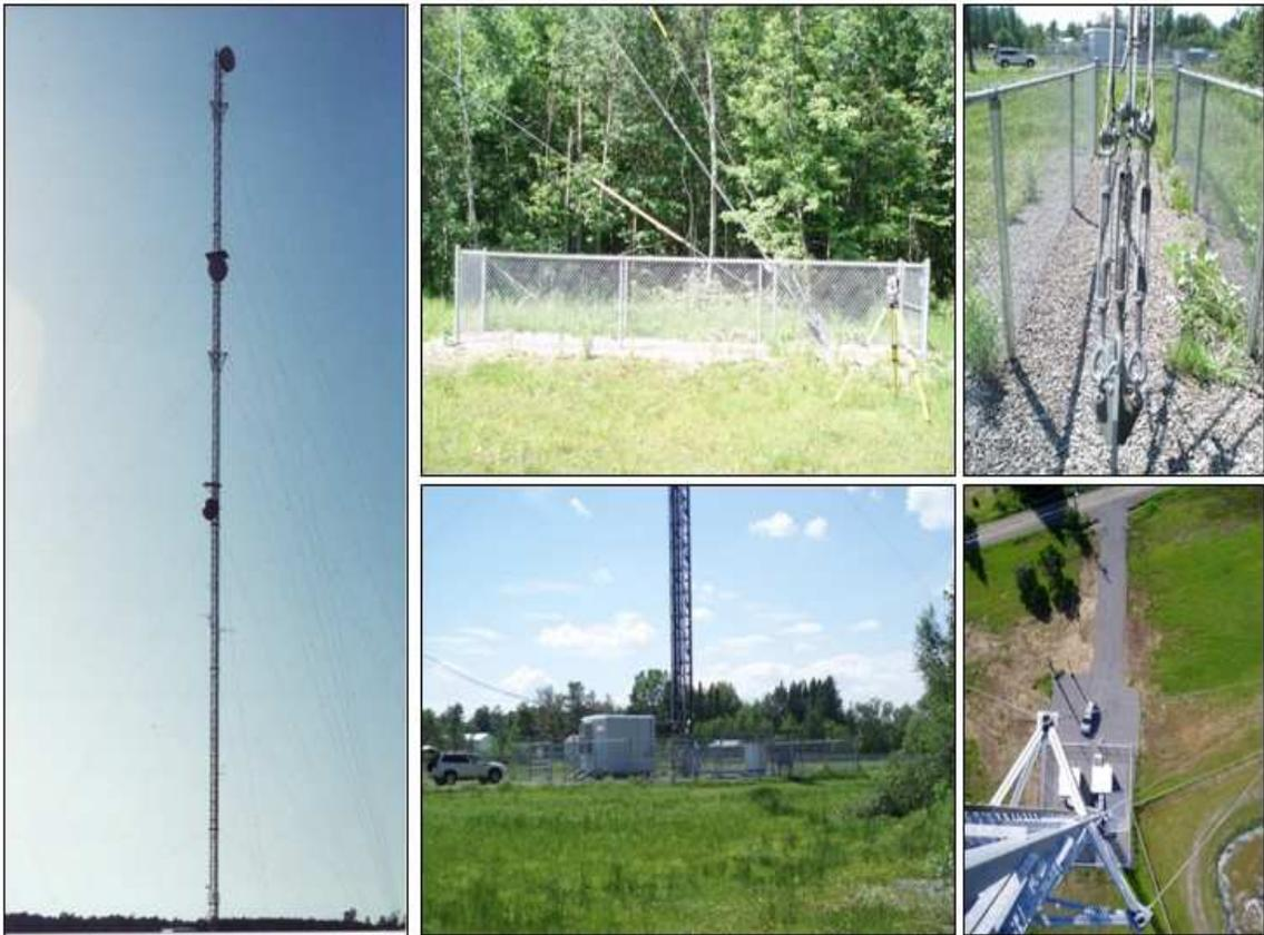
Figure 1-1. Example of a 111.2 m guyed telecommunication mast owned by Hydro-Québec in St-Hyacinthe, Québec, Canada.
