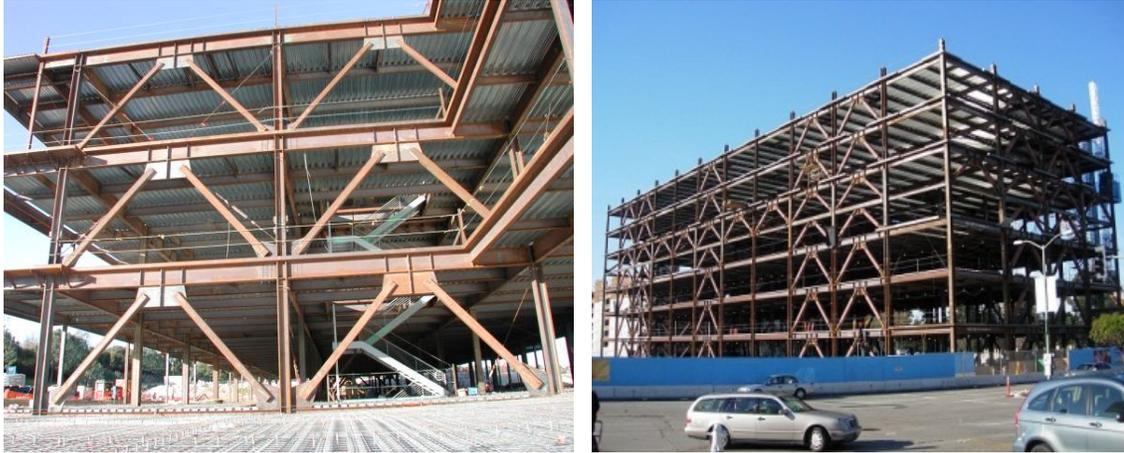
Figure 1.1 Examples of Concentrically Braced Frames (CBFs)
