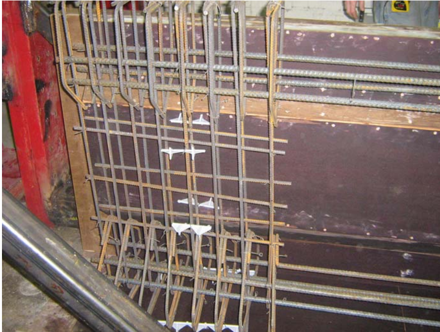
Figure 18: Details of reinforcing bars in end region
