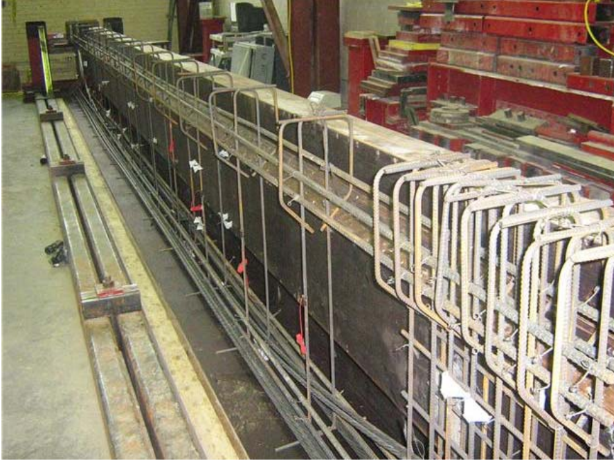
Figure 20: Details of stirrups and interface shear reinforcement
