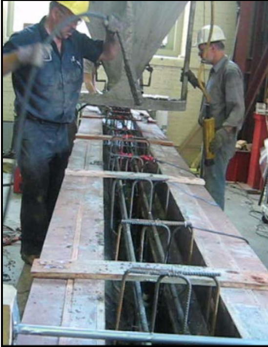
Figure 23: HPC girder casting operation
