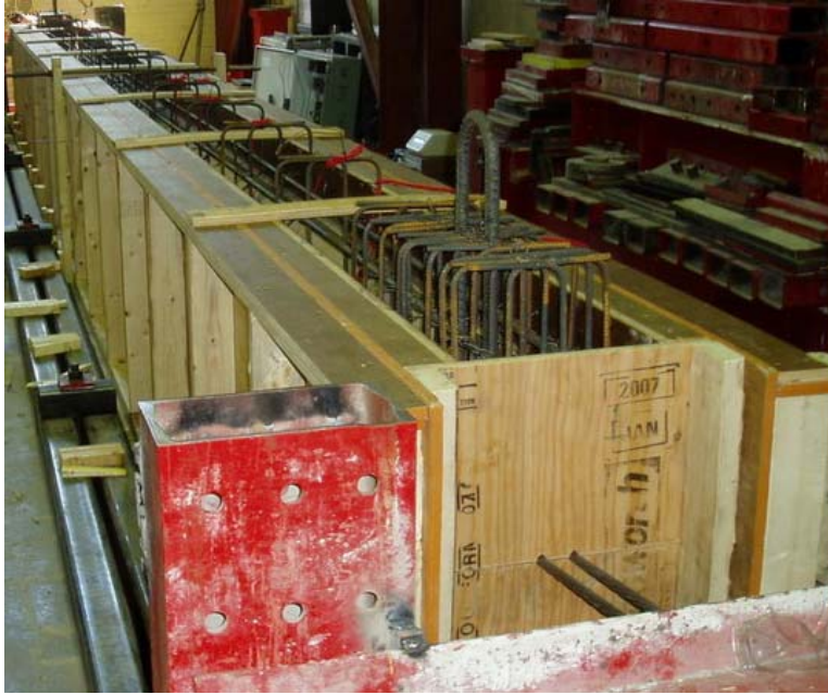
Figure 22: Reinforcing cage in formwork prior to casting
