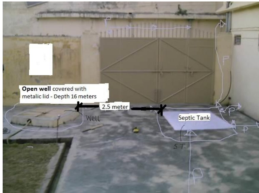
Figure 4.5: A typical septic tank and a dug well within the compound of a house in a town
