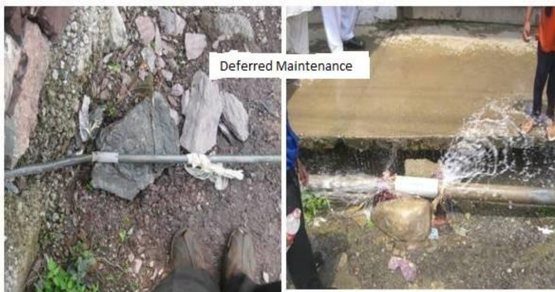
Figure 4.7: Wastage of water due to leakage and breakage, resulting from deferred maintenance
