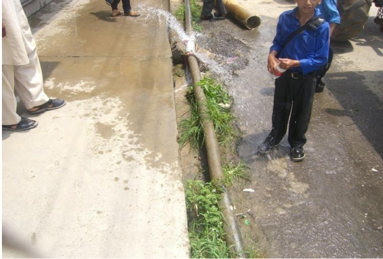
Figure 4.4: Condition of water pipe which is completely exposed in Mansehra
