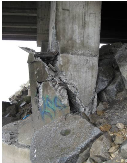
Figure 1.2: Shear failure of bridge column in the 2010 Chile Earthquake (Mitchell et al., 2011)
