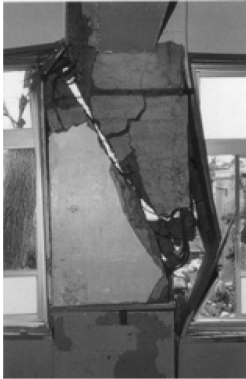
Figure 1.1: Damaged Column during 1995 Kobe Earthquake (Yoshimura and Nakamura, 2003)
