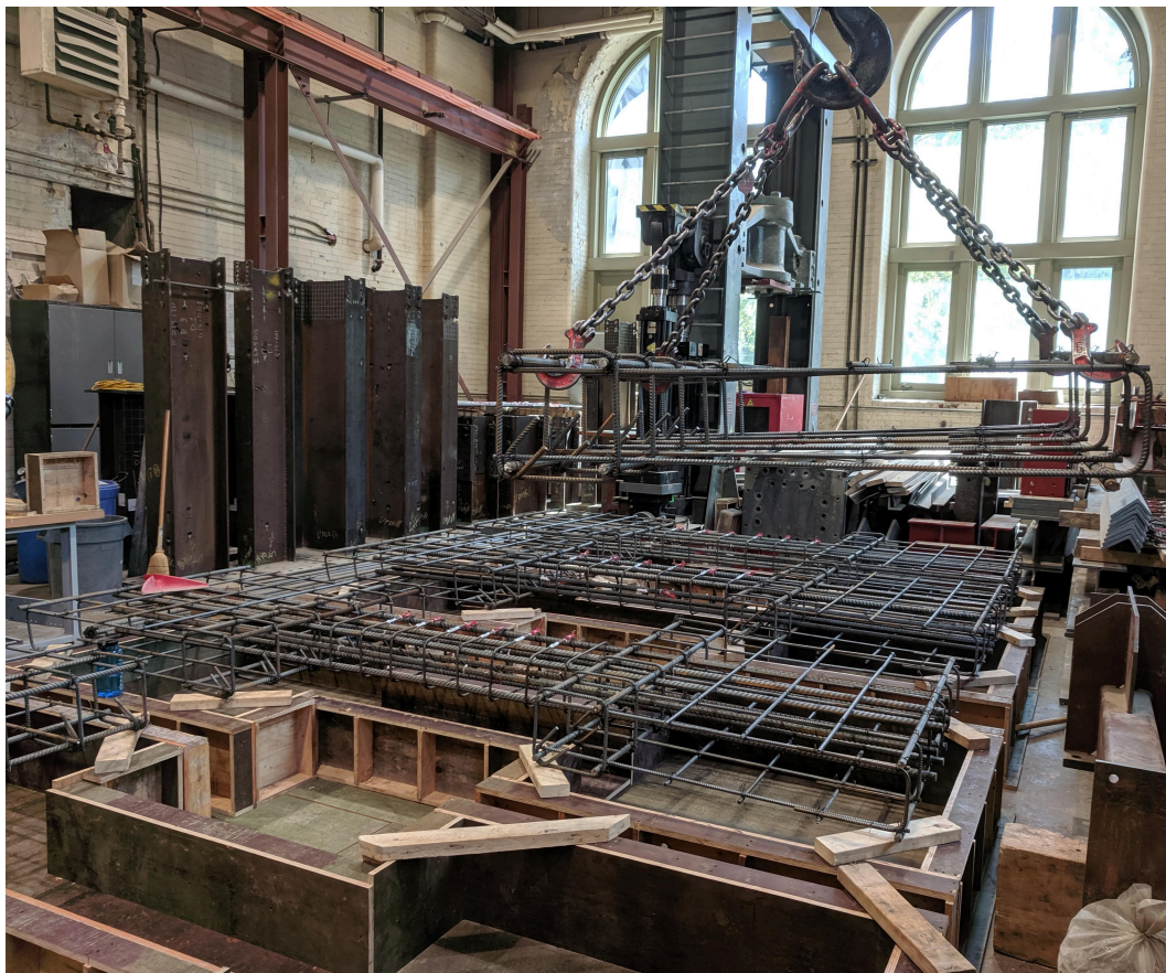
Figure 3.11: Placing of wall reinforcement cage above formwork for final assembly
