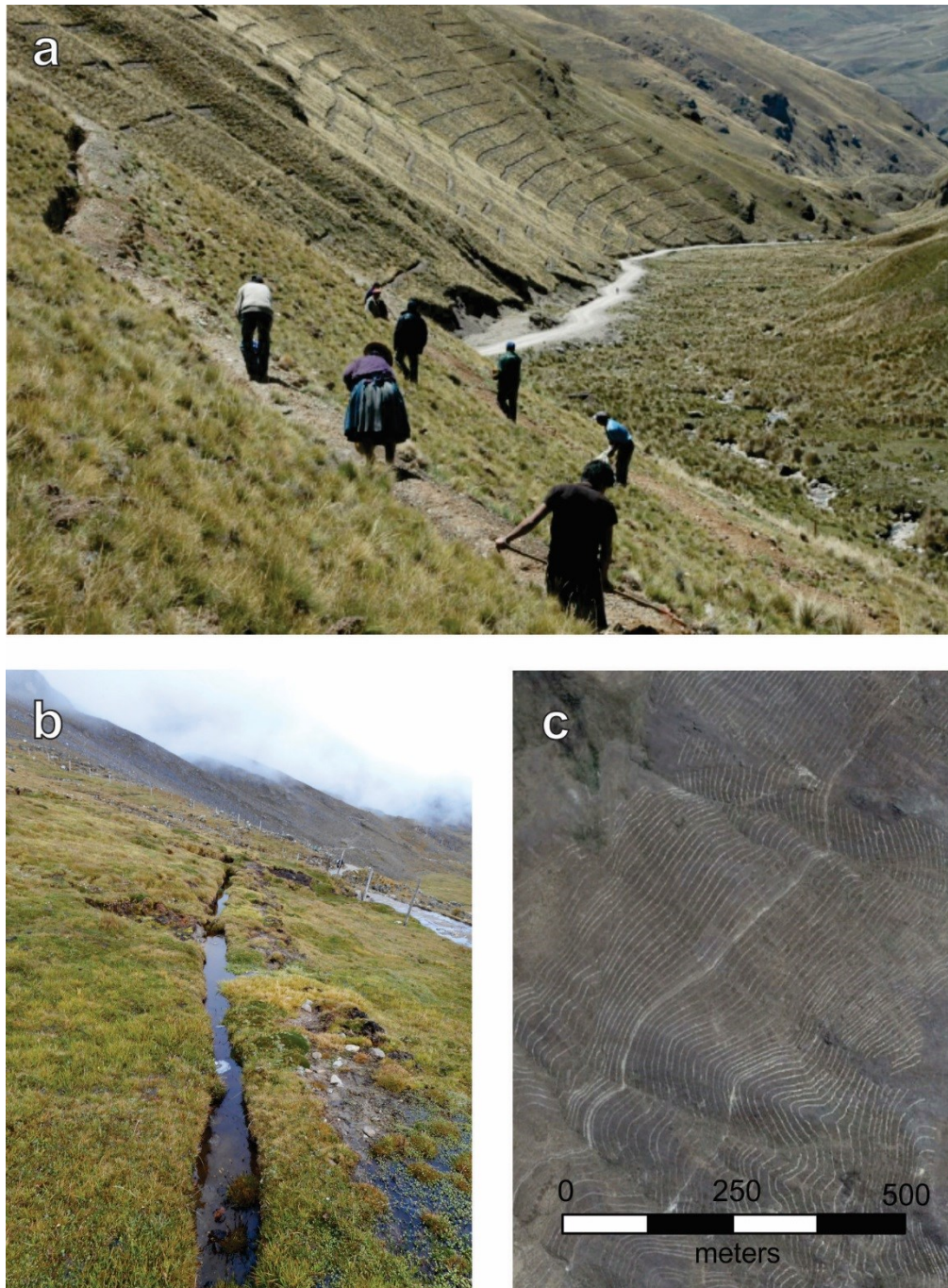
Figure 4.2: a. Construction of infiltration trenches as part of the World Bank and Care funded PRAA project. Photo taken from Comunidad Andina presentation; b. Infiltration trench with ponded water; c. Aerial view of trenched hillslope in the Shullcas Watershed, from Google Earth™
