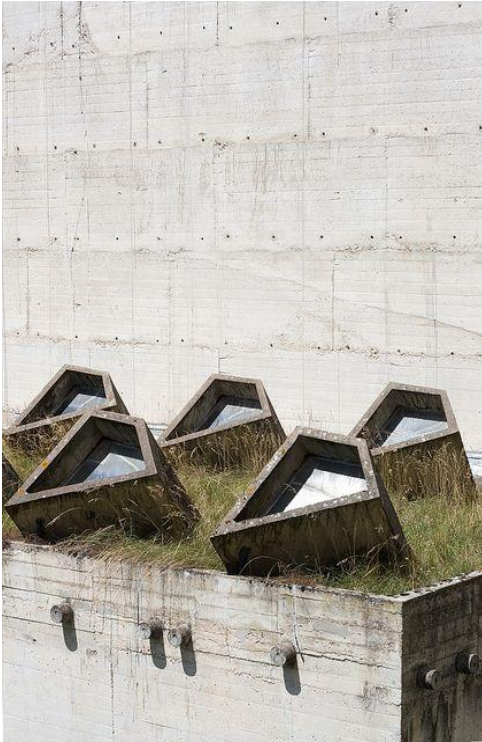
Figure 1.52 “Mitraillette” roof lights, La Tourette. From https://i.pinimg.com/originals/79/11/af/7911af8a0fa62e1eb5f2e1280436ca1a.jpg
