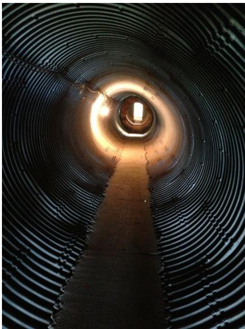
Figure 1.19 Tunnel at La Ribaute. Photograph by S. Wischer.
