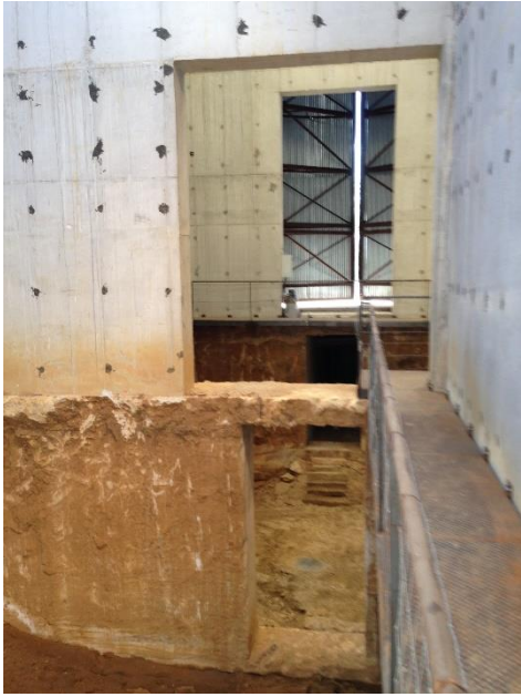
Figure 1.25 Interior walkway at La Ribaute. Photograph by S. Wischer.
