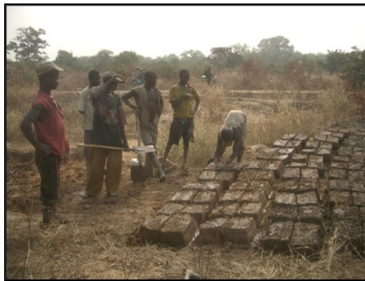
Figure 9.1: Brick-making for Construction of a Structure to House a Shea Nut Mill (Source: Author 2006)
