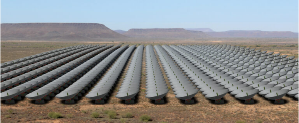
Figure 1.4: Rendering of future HIRAX array to be installed at the South Africa Radio Astronomy Observatory site in the Karoo. The array will consist of 1024 six meter parabolic dishes each with a single dual-polarization feed. Image credit Prof. C. Chiang.
