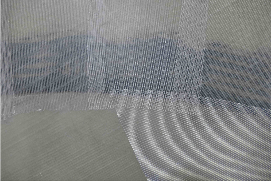
Figure 1.8: Mesh embedded inside surface of first D3A six meter dish.
