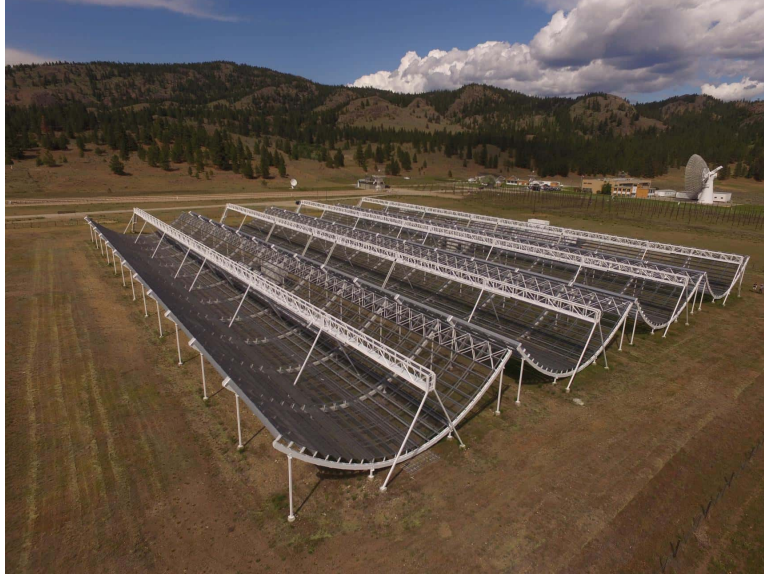
Figure 1.3: CHIME telescope located at DRAO near Penticton, BC. The telescope consists of four 20x100 m segments that each have 256 feeds. Photo from CHIME website [12].
