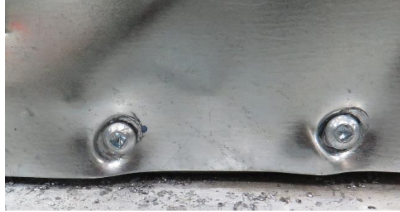
Figure 2.13 Sheathing steel bearing
