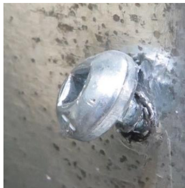
Figure 2.14 Sheathing screw tilting
