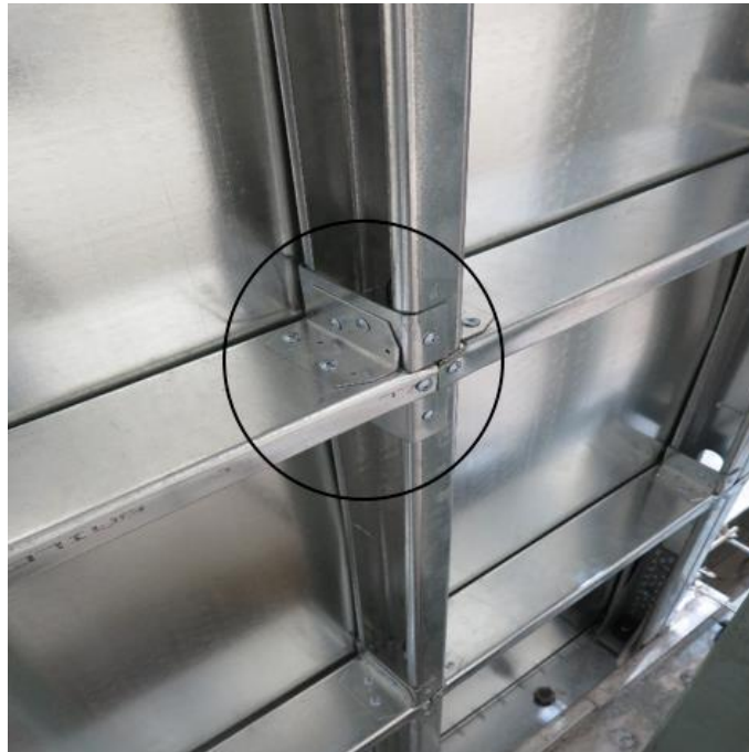
Figure 2.6 Blocking connection
