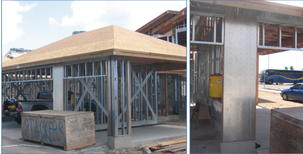
Figure 1.1 Cold-Formed Steel Wall Construction ( Courtesy of Jeff Ellis, Simpson Strong-Tie )
