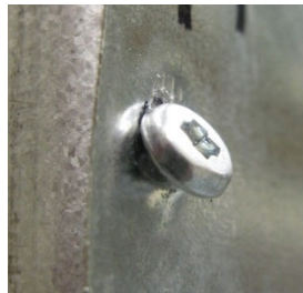
Figure 2.11 Sheathing Screw Tilting
