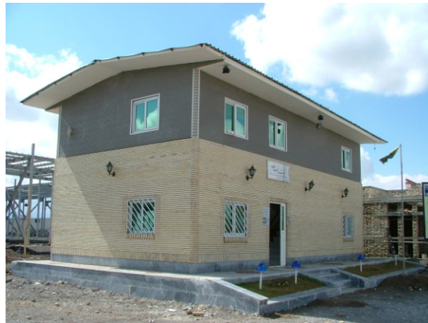
Figure C.46. The demonstration building built by the Rashestan Company.
