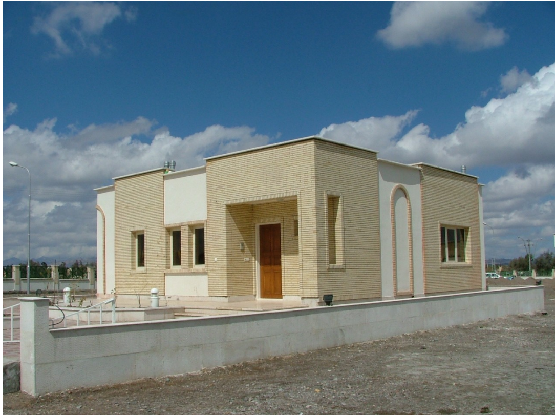
Figure C.18. The demonstration unit that HFIR has built at the exhibition site; the building uses its recommended construction method.
