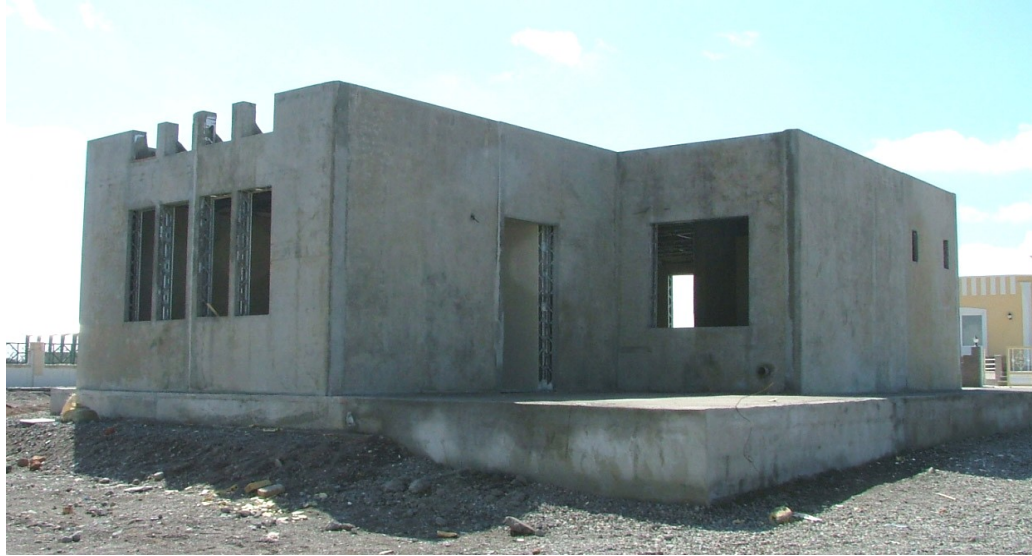
Figure C.37. The sand-cement plastered exterior of the demonstration unit built by MEHRSA Company.
