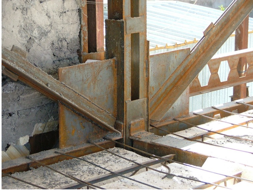
Figure 3.35. Over-designed framework of a two-storey house
