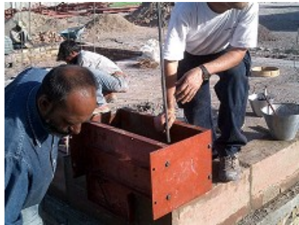
Figure C.43. Rammed earth blocks used for constructing the domed unit. Photo: PWJ
