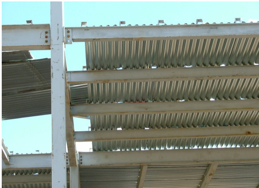
Figure C.15. Corrugated galvanized steel sheets are used as permanent shuttering.
