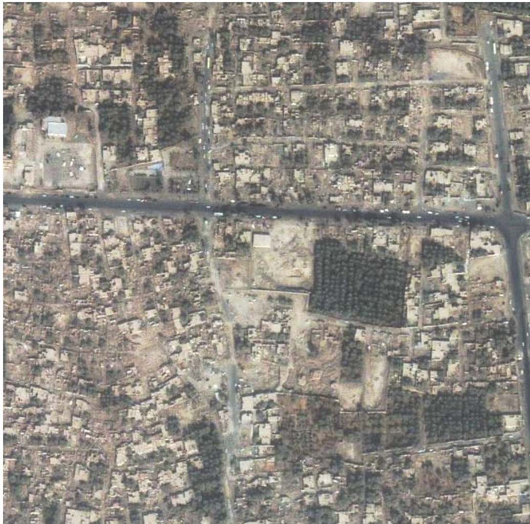
Figure 2.3. Close-up of the aerial photo of Bam one day after the quake. The collapsed roofs of both old and new houses can be seen. The upper section of the photo shows the old fabric while the lower part is mostly composed of relatively new constructions (IKONOS 2003), IKONOS Image Courtesy of GeoEye
