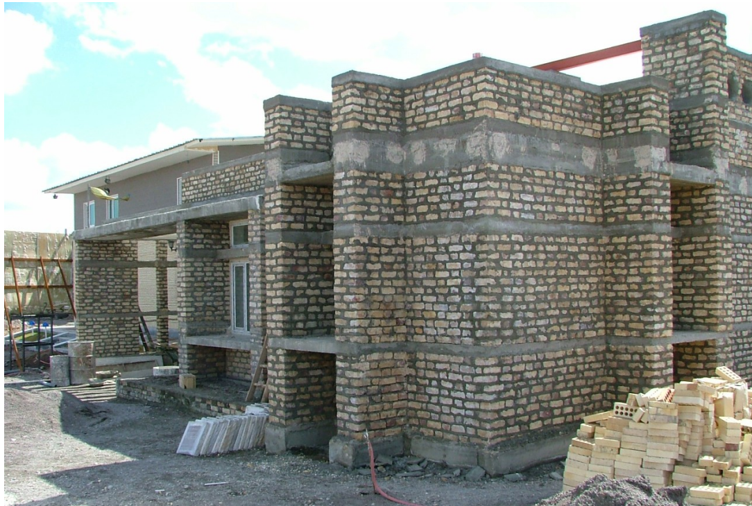
Figure C.44. The demonstration house that PWJ was building at the time of visit. The four horizontal reinforcements (ring beams) are clearly shown in the picture.
