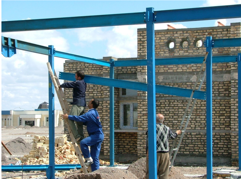
Figure C.11. The structure of a 9x9 m 2 house can be installed in its place in few hours by only two labourers.
