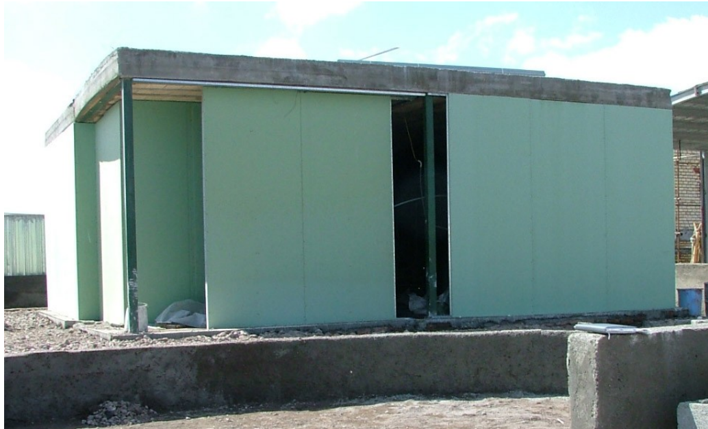
Figure C.29. The sample house built at the exhibition site by Azar-Mahd Construction Company. The house was not finished at the time of visit.
