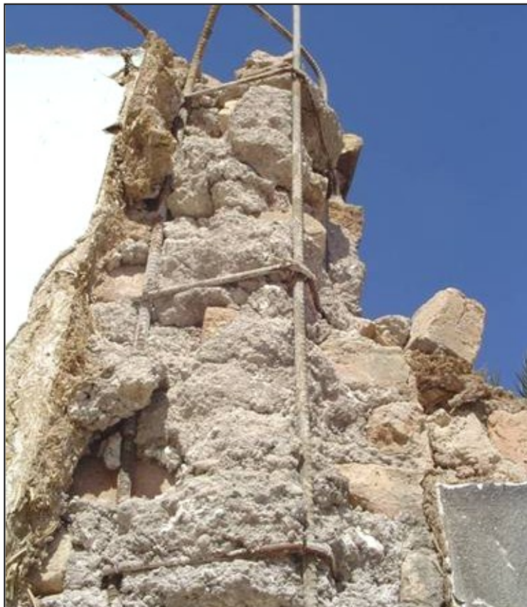
Figure 3.15. Poor quality of concrete indicates lack of concrete construction know-how. Photo: HFIR archive
