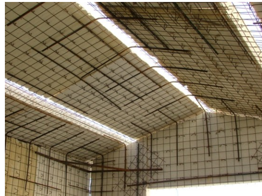
Figures C.21, C.22. Reinforcements are created in the corners as well as other critical joints by additional steel bars.
