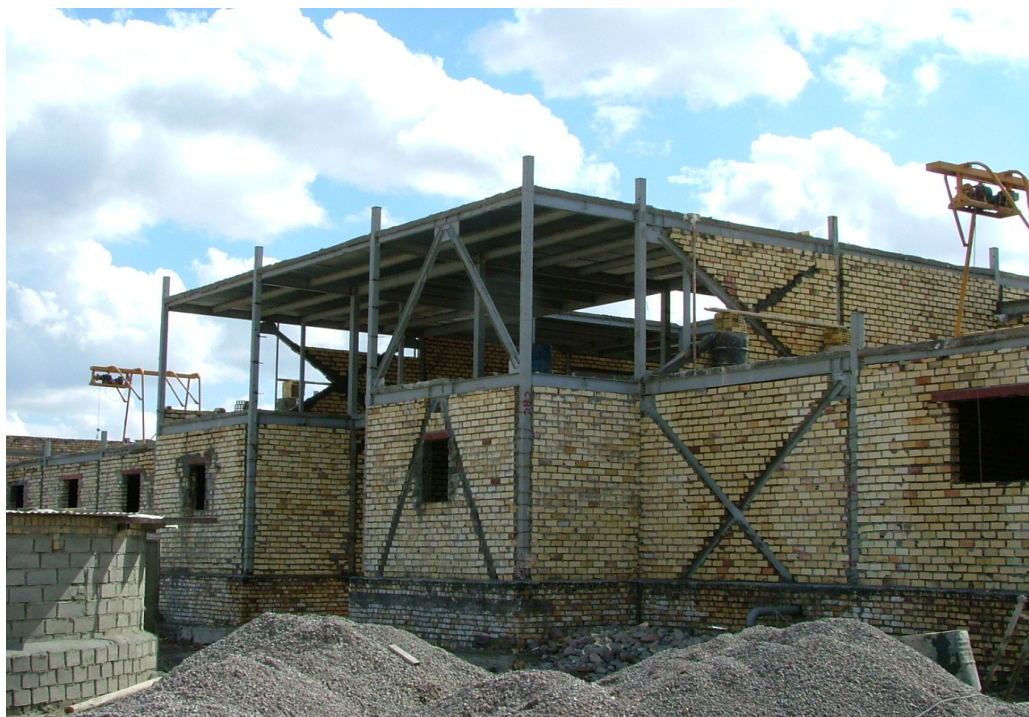
Figure C.12. A publicly funded building being built by HFIR, employing its recommended structural elements.
