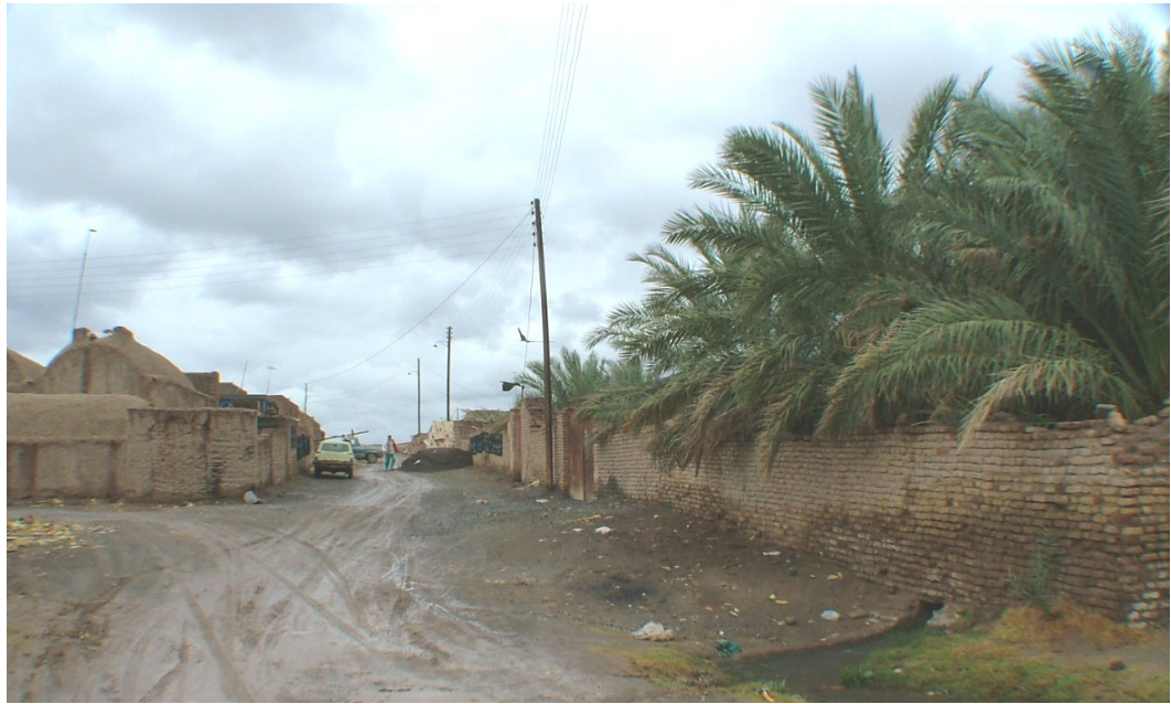
Figure C.53. A view of Kûrk showing its vernacular architecture and landscape.
