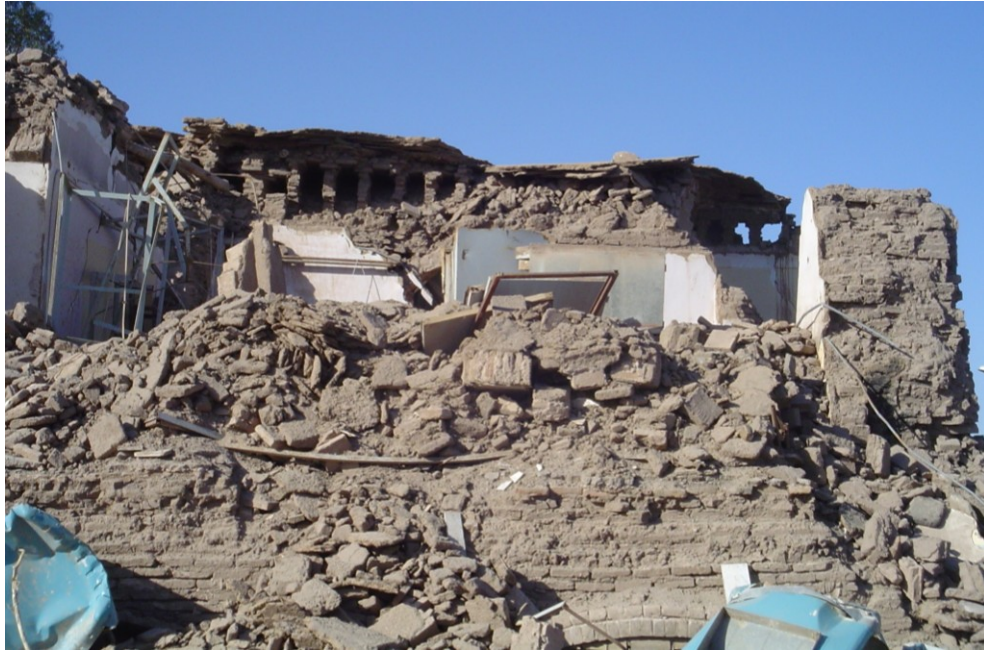
Figure 3.2. Placing reinforcements in load bearing walls is not common practice in Bam. Photo: HFIR archive
