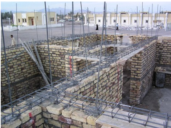
Figure C.41: The third ring beam is being prepared for the pouring of the concrete. Photo: PWJ
