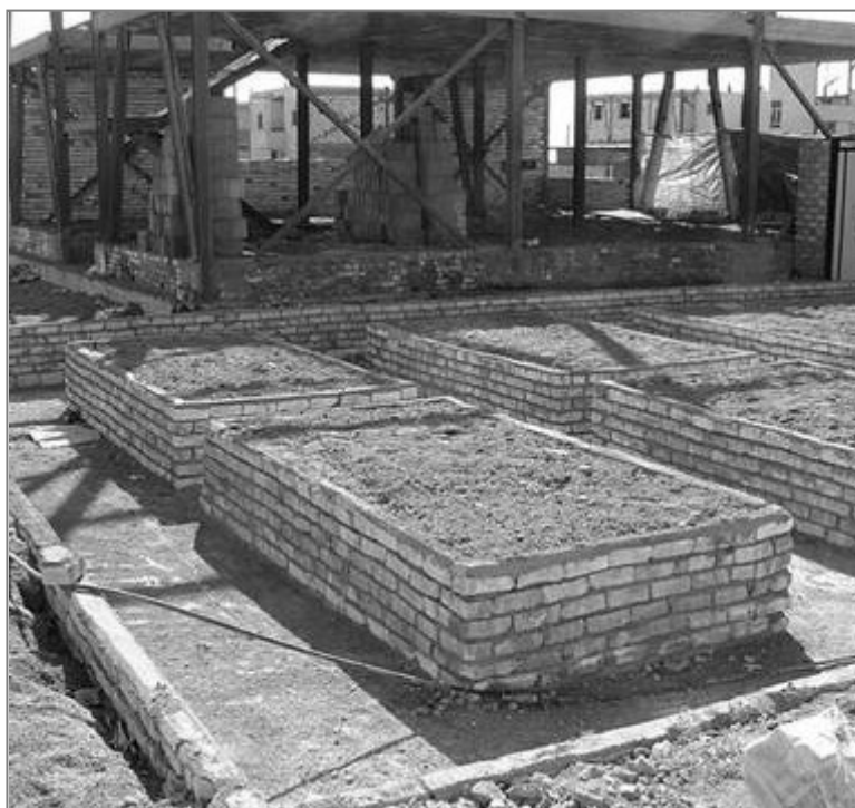
Figure 3.31. Foundation formwork made of brick walls
