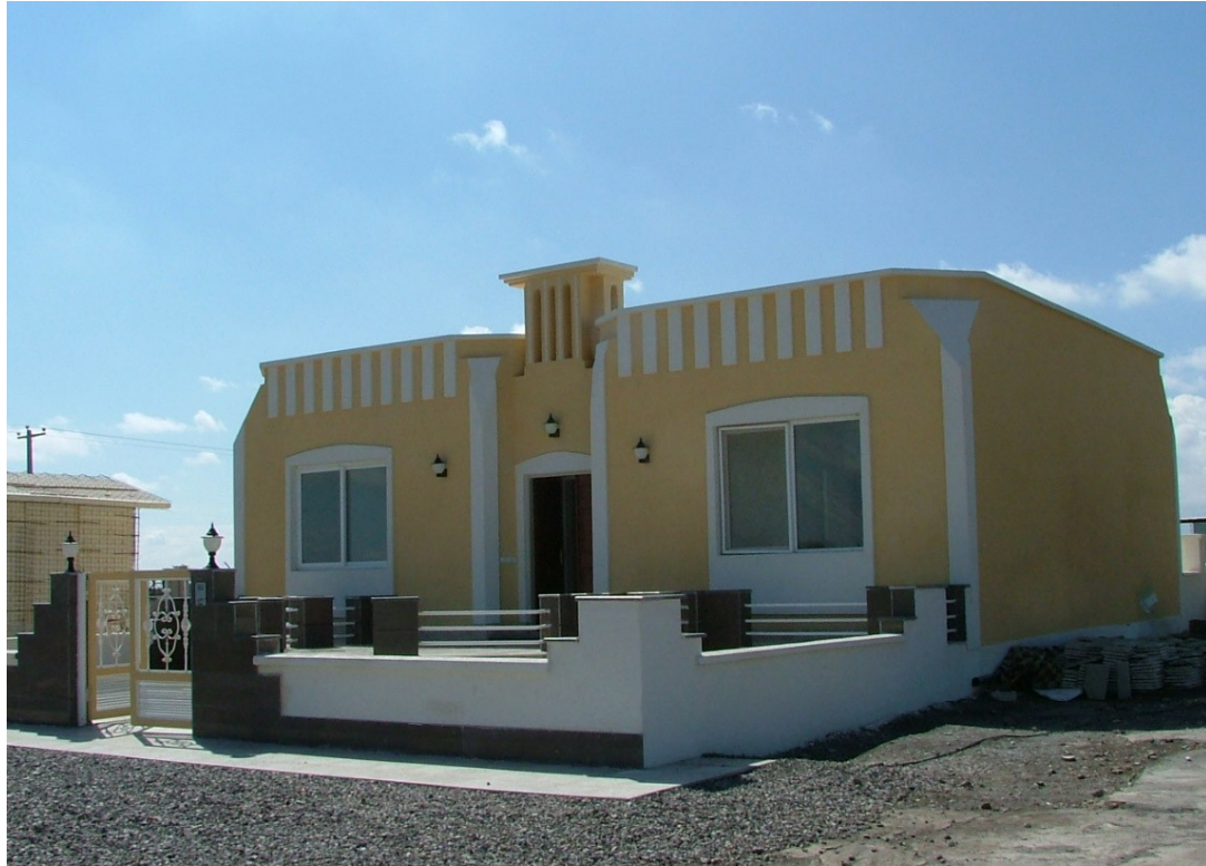
Figure C.23. The demonstration house built out of sandwich panels by BBOI at the exhibition site.
