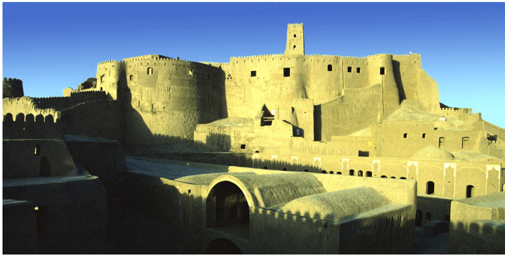
Figure 2.1. Bam citadel before the earthquake, one of the biggest earth complexes in the world
