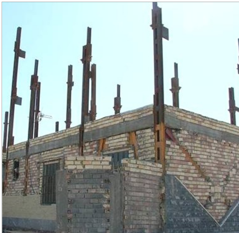
Figure 3.38. Columns extended above the roof line, ready for the future extension of the house
