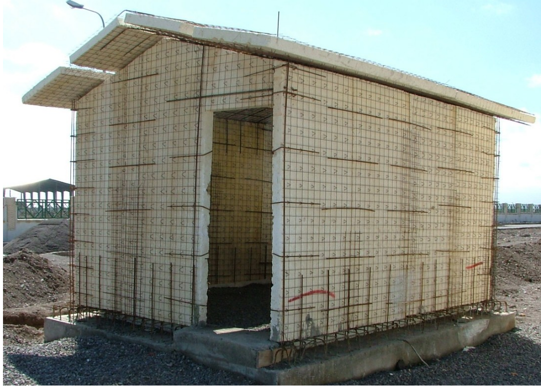
Figure C.20. The hut built of sandwich panels, left incomplete to show the construction details to the locals.
