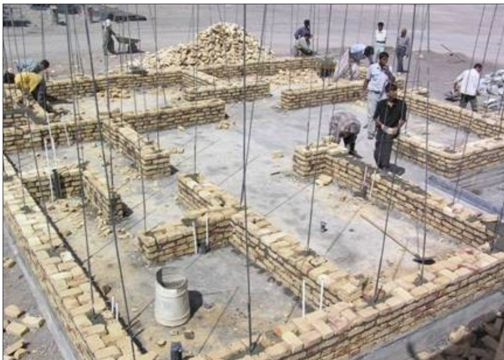
Figure 3.30. Vertical reinforcements. Photo courtesy of Peace-Winds Japan
