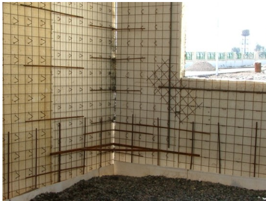
Figures C.21, C.22. Reinforcements are created in the corners as well as other critical joints by additional steel bars.
