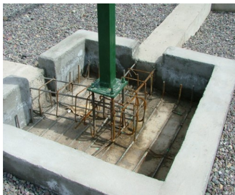
Figures C.7, C.8, and C.9. The structure designed and recommended by HFIR, left incomplete at the exhibition site to teach the local population how to implement this method.
