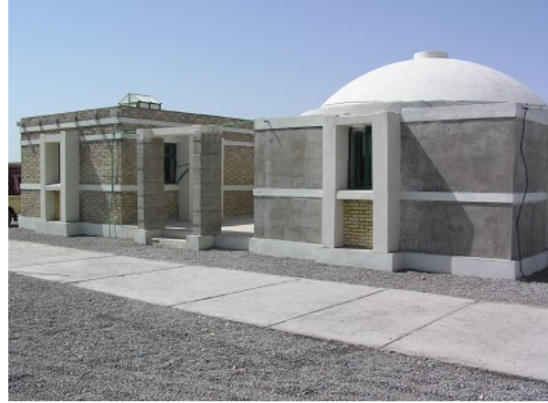
Figure C.42. The two office units PWJ has built for the use of HFIR. Photo: PWJ
