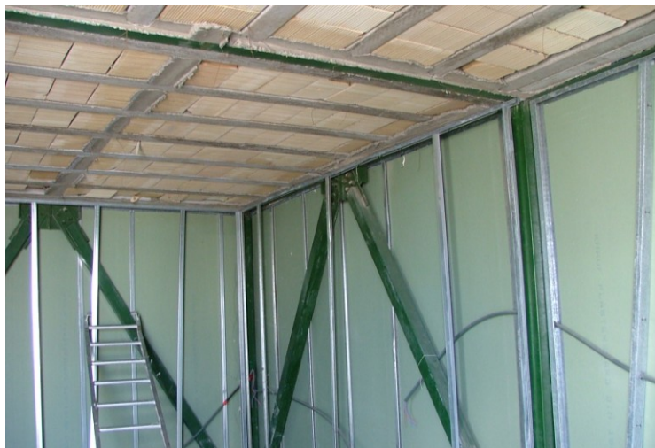
Figure C.28. The block-joist roofing system and drywall on steel studs
