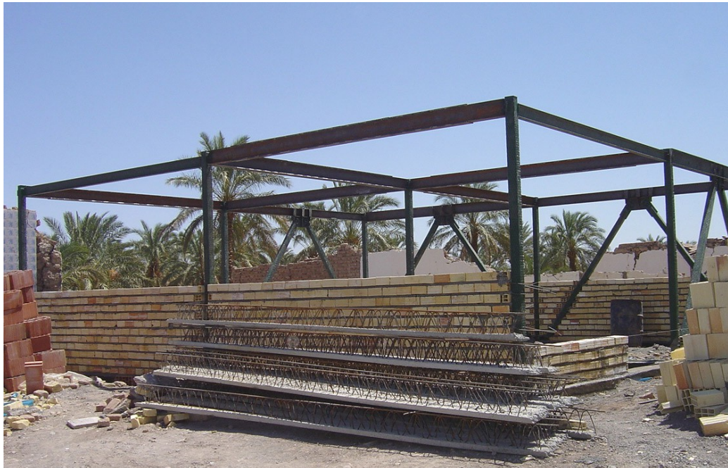
Figure C.17. The wall infill and roofing system may change from the HFIR recommendations. Here, hollow blocks were used as wall infill and a joist-block roofing system was employed. Photo: HFIR archive
