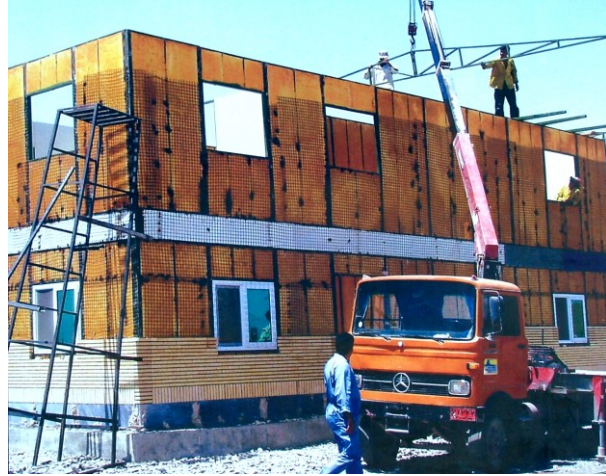
Figure C.45. Prefabricated triple Howe trusses installed in the place by a crane.
