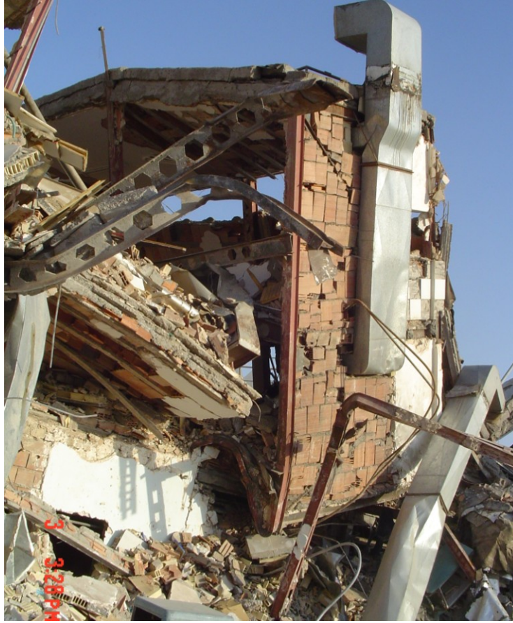
Figure 3.5. Inadequate design and weak steel profiles have turned the entire building to rubble. Photo: HFIR archive
