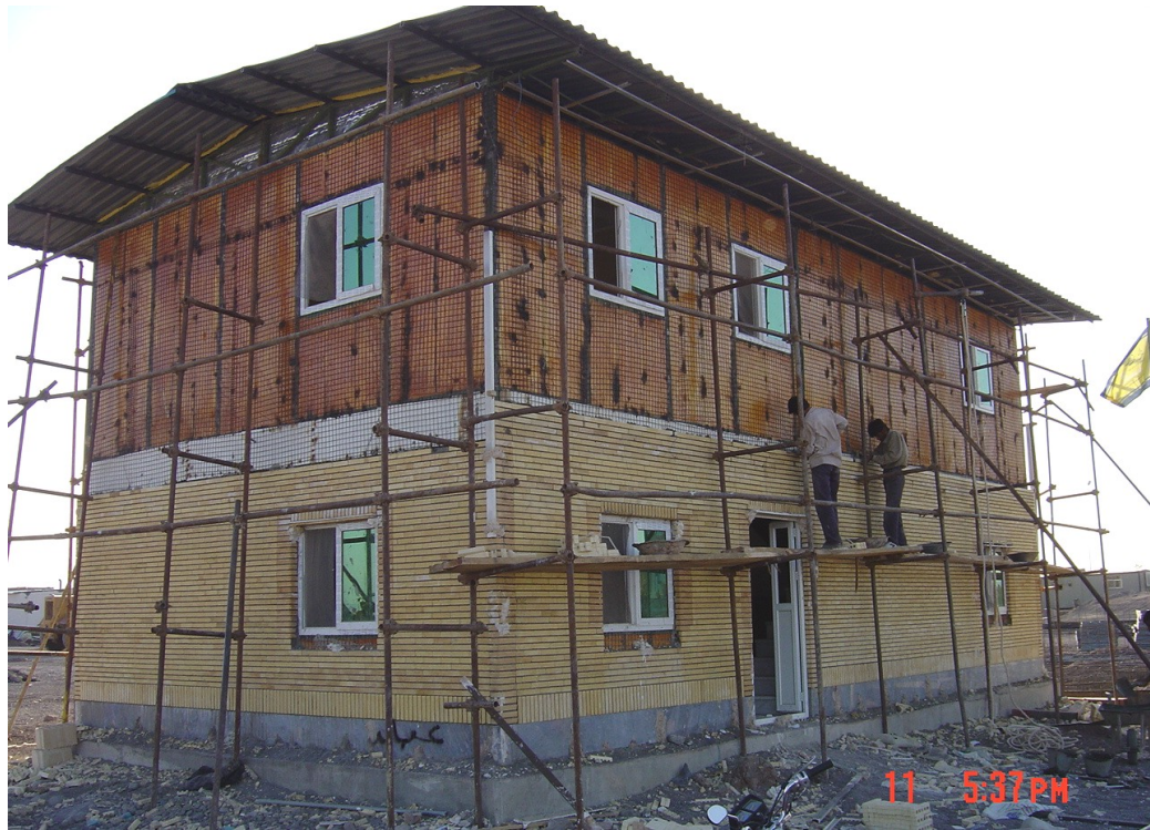
Figure C.47. The façade is being covered with slim façade bricks. The steel mesh makes a good bond between the façade bricks and sandwich panels. Photo: HFIR archive
