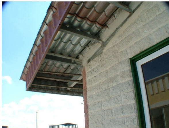
Figure C.26. Corrugated steel sheet on Z-shaped girders.
