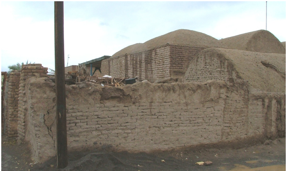
Figure C.49. The vernacular architecture of Kürk consisted of adobe load bearing walls and barrel vault roofs.
