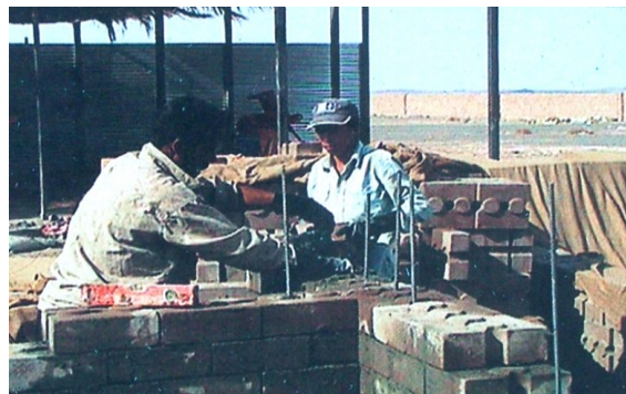
Figures C.30, C.31. Interlocking CEB and inter-wall reinforcements
