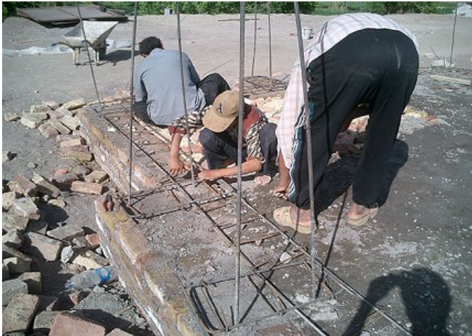
Figure C.40. Implementing the first ring beam at the plinth level. Photo: PWJ
