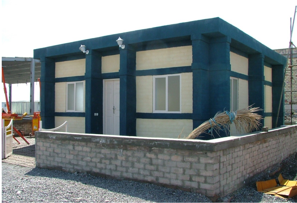
Figure C.33. The house built cooperatively by Auroville and the International Blue Crescent, using CEB and vertical steel bar reinforcements along with ring beams at three levels: sill, lintel, and roof.
