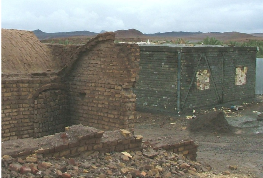
Figure C.51. The new house took the place of the courtyard. The windows of the new house were bricked due to the climatic problems they created.
