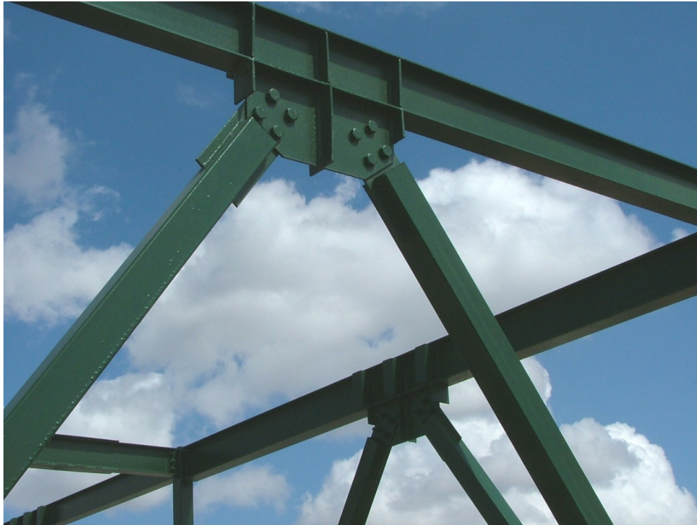
Figure C.10. The structural system proposed by HFIR can be easily and quickly assembled with bolts.
