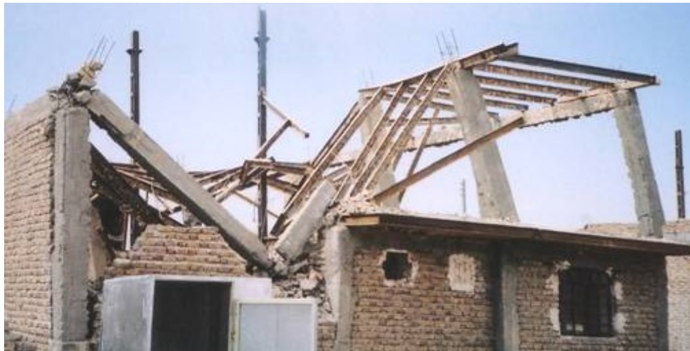
Figure 3.17. Incompatibility of materials in hybrid building results in the reduction of strength. Photo: ISEO 2004
