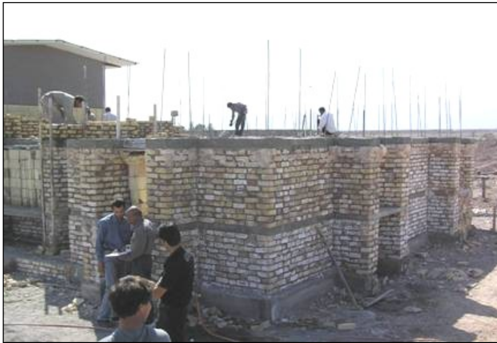
Figure 3.29. Horizontal reinforcements (ring beams) Photo courtesy of Peace-Winds Japan
