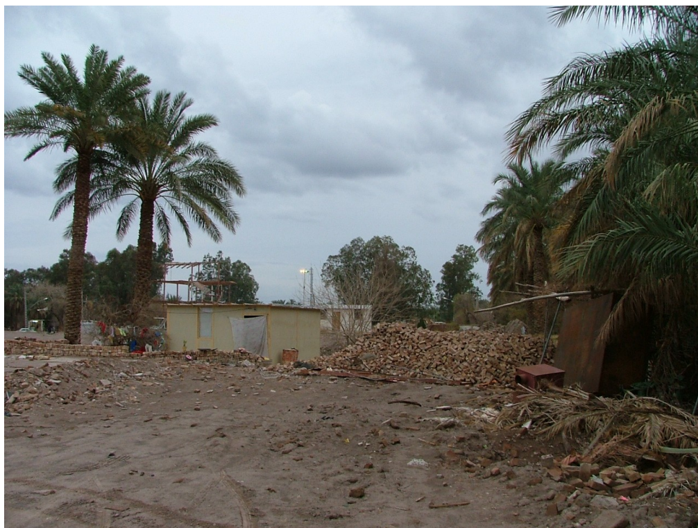
Figure C.4. Many families still lived in containers or other types of temporary accommodation, such as first-aid tents in a few cases.
