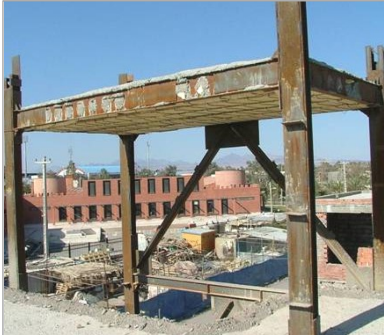
Figure 3.39. An oversized structure: there is little load to bear, yet the posts are highly reinforced; double I-beams are welded together, reinforced by a longitudinal steel plate welded all the way to the two beams
