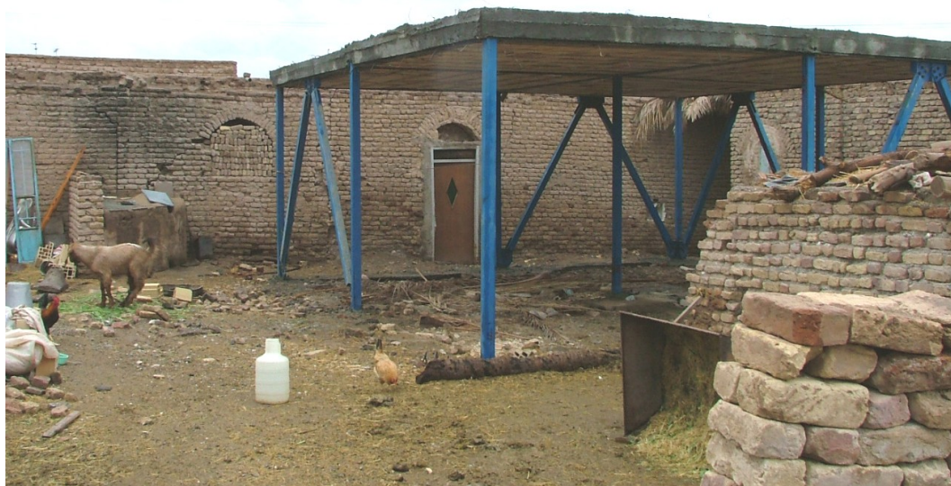
Figure C.50. HFIR is constructing new houses in the existing courtyards of the old houses of the villagers.
