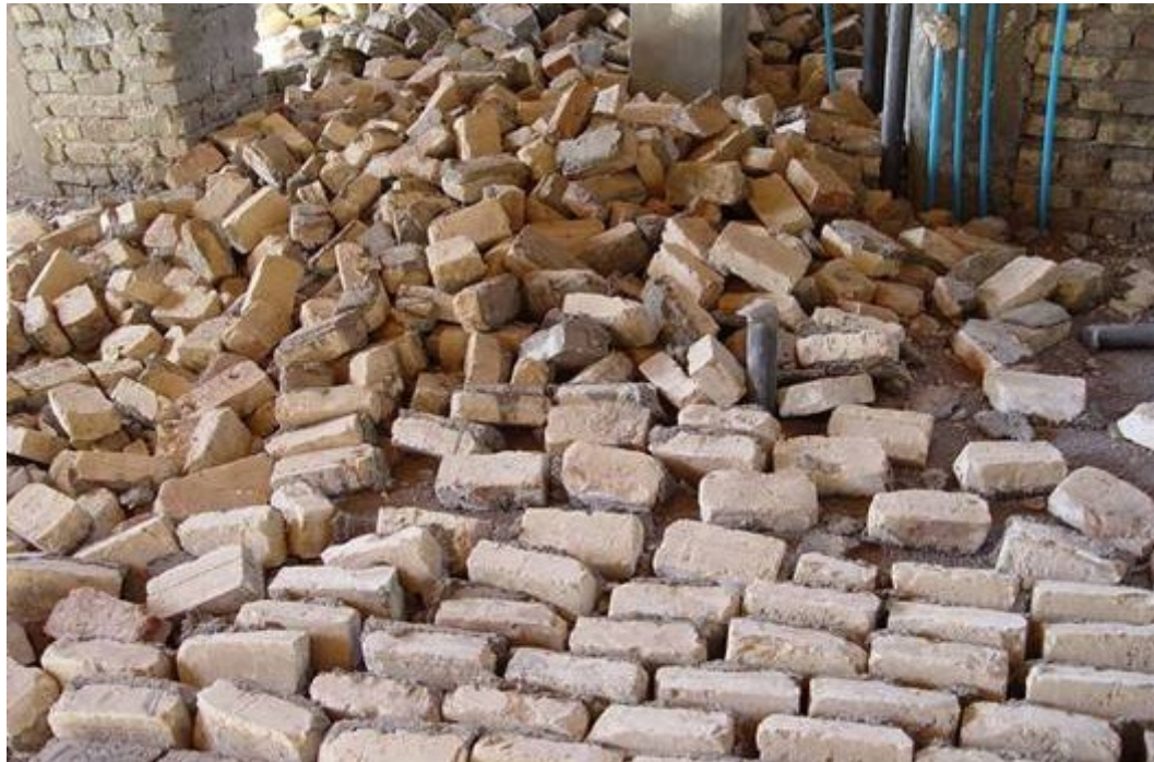
Figure 3.19. When bricks are laid without being soaked, they make a very weak wall. Photo courtesy of Peace-Winds Japan
