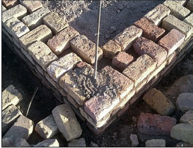
Figure C.39. Steel bars placed within the walls as vertical reinforcements Photo: PWJ
