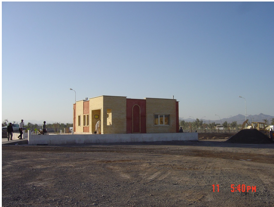
Figure C.6. Each construction company could build a demonstration unit showcasing its proposed method. Photo: HFIR archive
