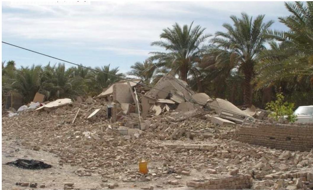
Figure 3.1. Lack of a decent foundation was a common problem among the buildings destroyed in Bam. Photo: ISEO 2004
