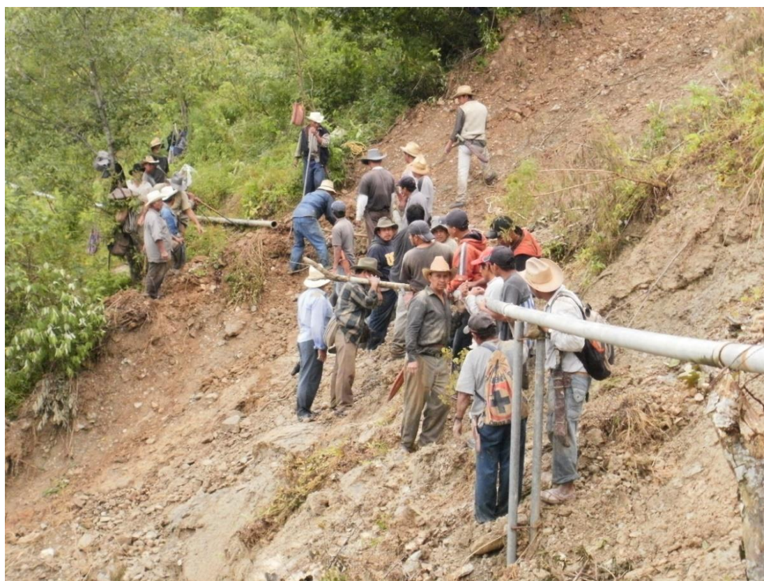
Image 32. Water committee assessing and temporarily repairing damaged water network in 2010. (Photo, Leonardo Ávalos Bis)
