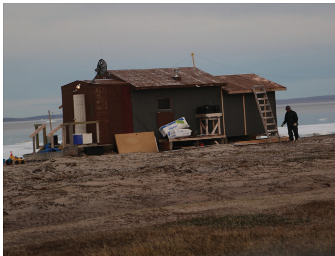
Figure 182. Fully electrified cabin on the coast, connected to a generator and satellite dish.
