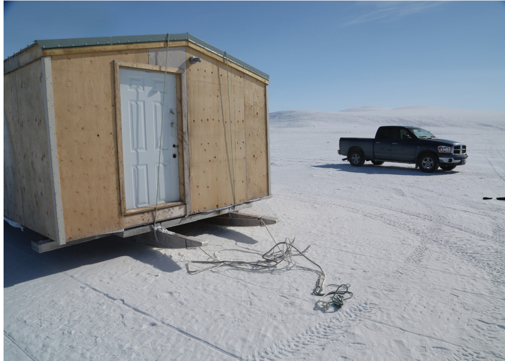
Figure 146. New cabin built in town and about to be hauled to a campsite at Clyde Inlet.
