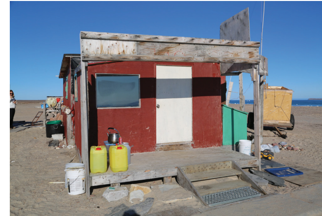
Figure 134. Red cabin with a sideview entrance facing south and a wind-catcher to sweep snow from the front door.
