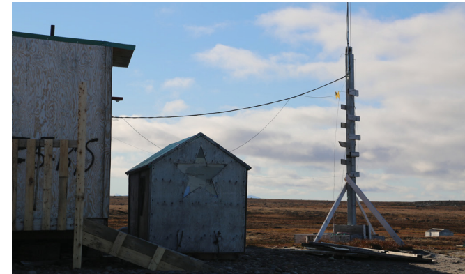
Figure 164. Post serving as an antenna, electrical post, and signage to named places along the coast.
