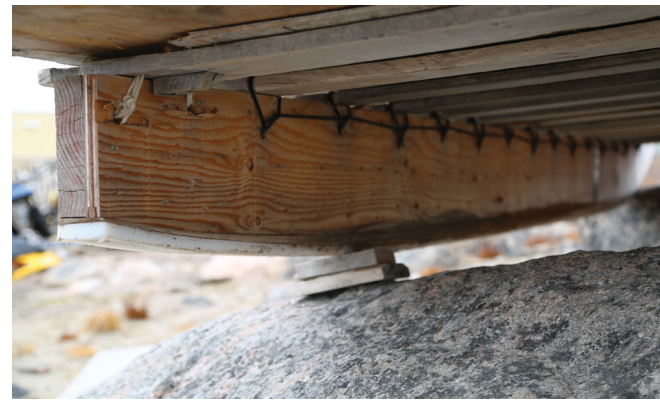
Figure 181. Teflon strips to minimize friction.
