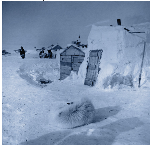
Figure 64. Beginning of a hybrid construction era, Resolute Bay, NWT (Lunney, 1956a).
