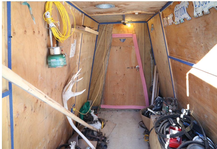
Figure 116. The interior of the tuqssuk added for additional storage and keeping the cold air out of the workspace.
