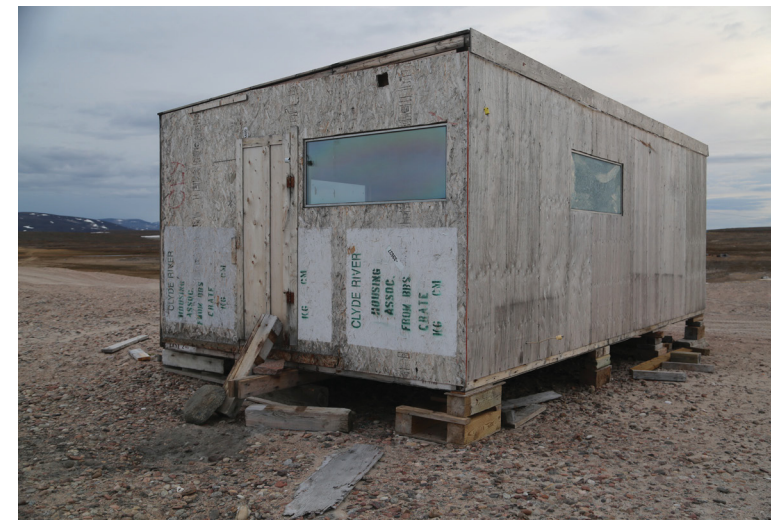
Figure 159. Plywood cabin resting comfortably on plywood crates, with an unobstructed view of the ocean.
