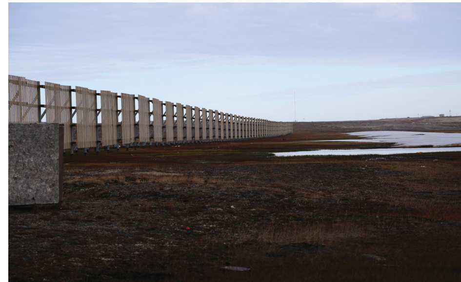
Figure 157. The windscreen built for $2,000,000 to prevent snow from drifting across the main road to the airport and from blocking the main entrance to the cultural school in Clyde River.
