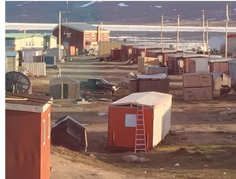
Figure 108. Seacans or containers, trailers new and old, sheds, old vehicles, dog houses, boats and fishnets added porches and outbuildings occupy the gap spaces.
