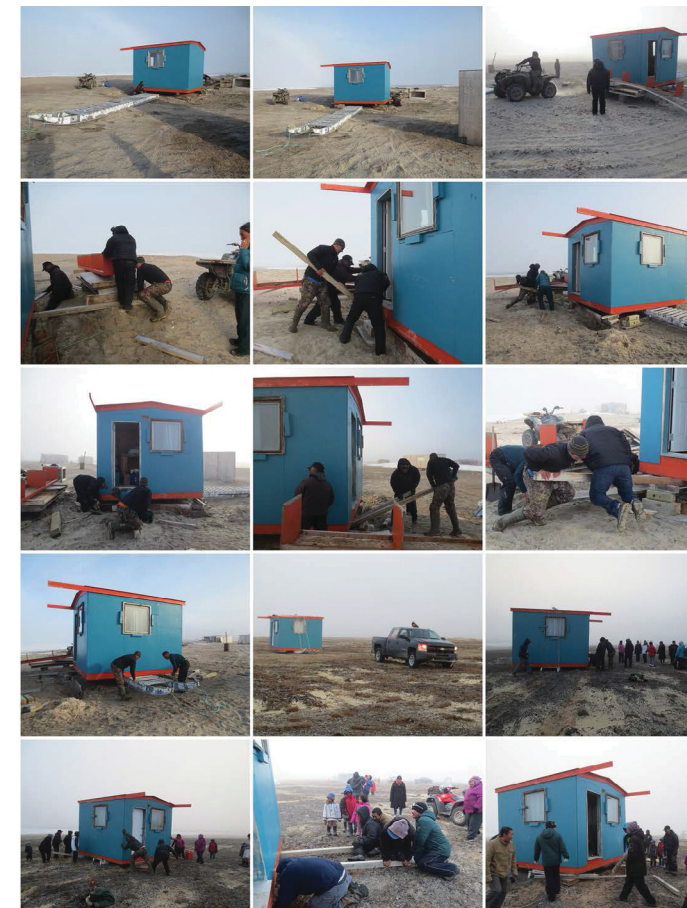
Figure 131. It takes a community to haul a small cabin during the summer (Gearheard, 2015). Hauling on the sand requires a four-wheel truck, a strong qamutiiq, and some quick thinking.
