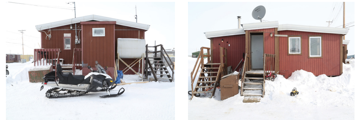
Figure 113b. If the original government house has a porch and entryway that is appropriately oriented, it is usually so small, people would leave the front door opened to facilitate access.
