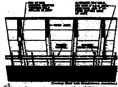
Fig. 4.43 Suspended ceiling constructed with metal runners and lath. (Source: Hawkins & Abbe, 1948)
