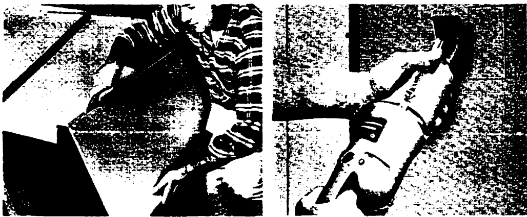
Fig. 4.38 Wallboard was developed to be cut with a knife or saw. Left: cutting the board with a knife. Right: cutting the board with a power saw. (Source: Wagner, 1976)
