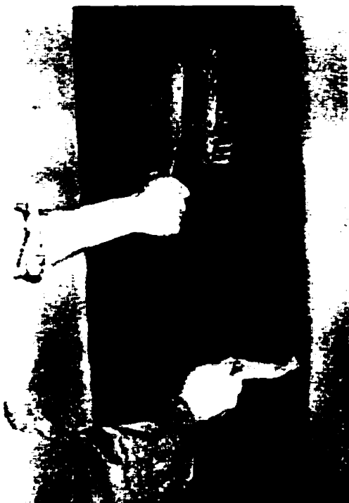
Left: Fig. 4.30 A crude method of painting before the 1940s: to get a satisfactory surface texture, it was better for two people to work together, one to distemper while the other used the stippling brush on the freshly distempered wall. (Source: Molloy, 193-?)
