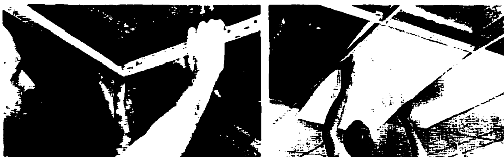
Fig. 4.46. Installing cross-tees between main runners. (Source: Wagner, 1976)
