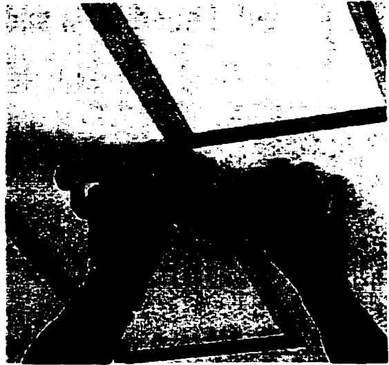
Fig. 4.51 By the use of innovative furring tapes, tiles can be directly installed on drywall ceilings. (Source: Armstrong, 1999)
