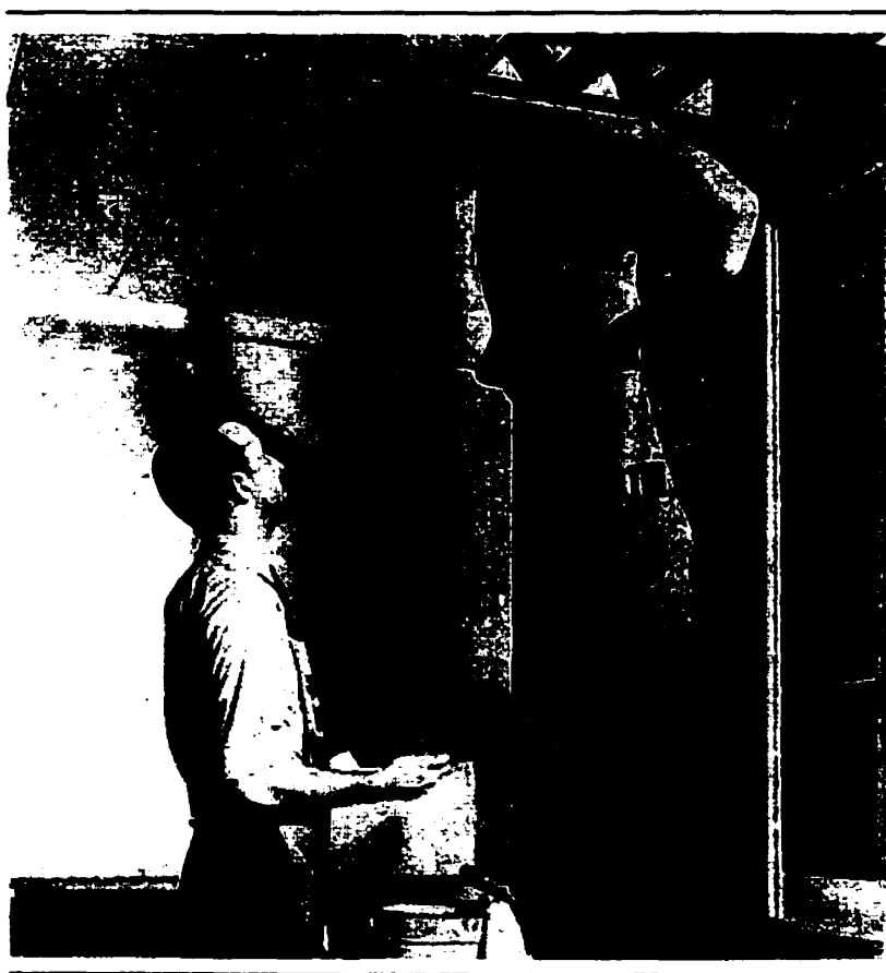
Fig. 4.44 Attaching fiberboard tile with adhesive. (Source: Hawkins & Abbe, 1948)
