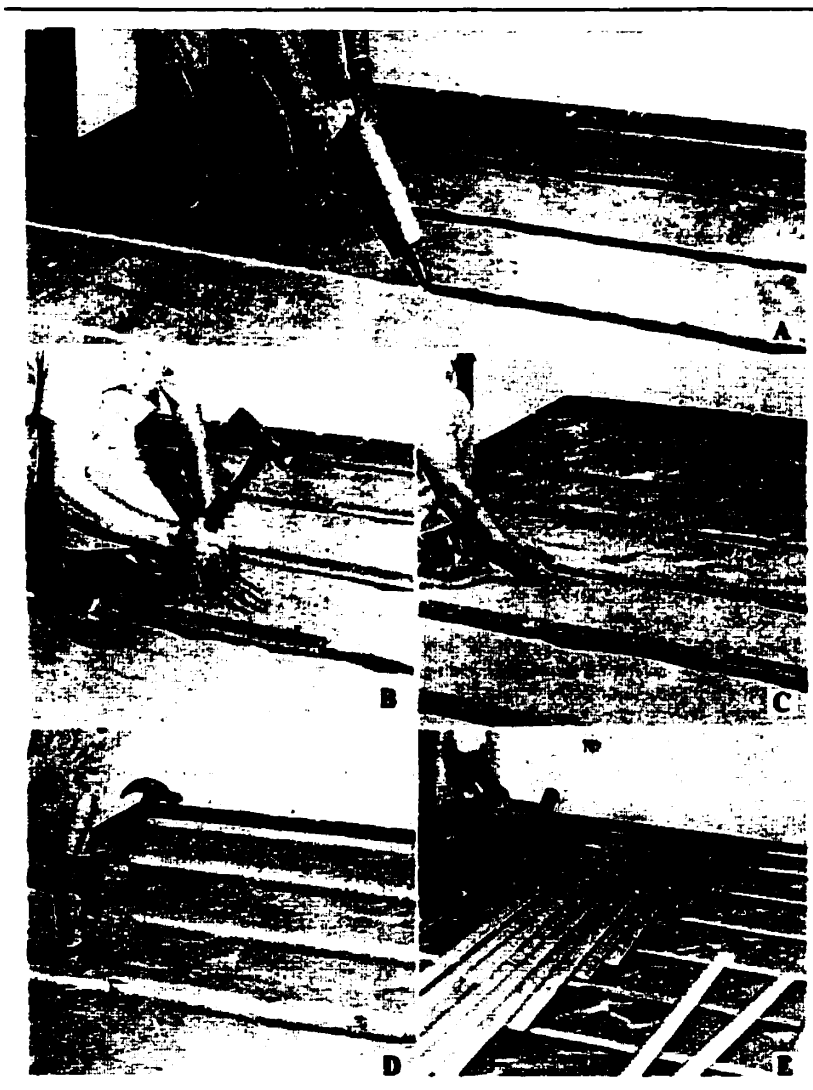
Fig. 4.26 Installing strip wood flooring over concrete slab: A: applying rivers of mastic along layout lines. B: nailing bottom strips in space. C: spreading polyethylene film over bottom strips. D: nailing top strips to bottom strips. E: nailing strip flooring to sleepers. (Source: Berkeley, 1968)
