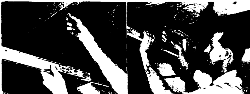
Fig. 4.45 Left: installing screw eyes in a joist to support metal runners. Right: tying a runner to a screw eye with wire. (Source: Wagner, 1976)
