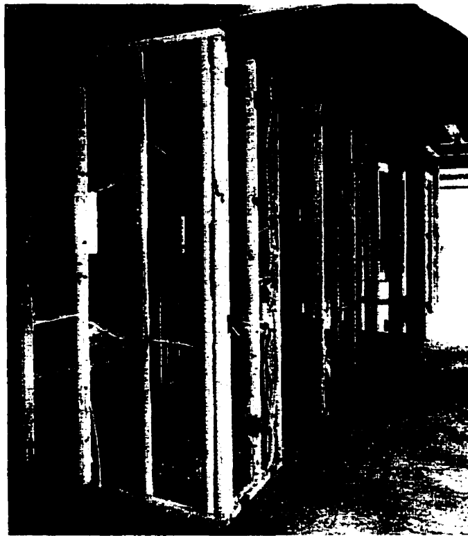
Fig.4.9 Wiring goes through holes in the studs of interior partition walls. (Source: Benson, 1997)
