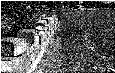
Edgewater Park BEFORE (looking east)
