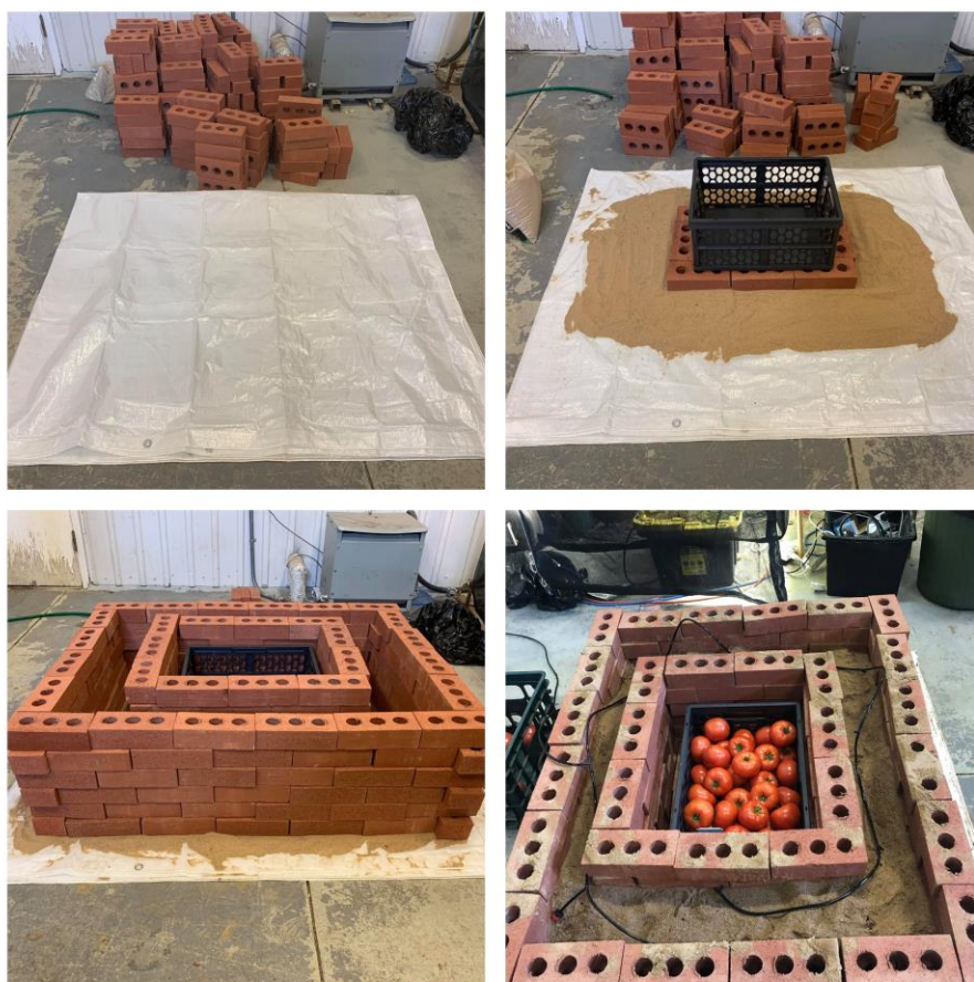
Figure 2. Construction process of the RCB Evaporative Cooler
