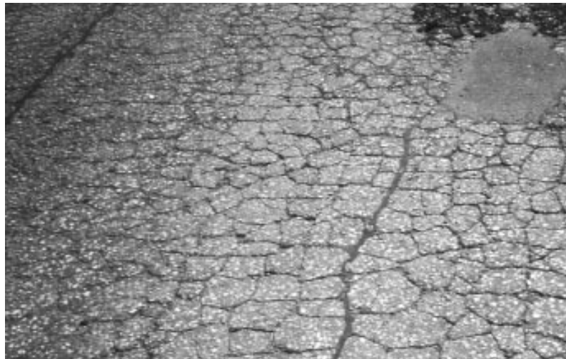
Figure 2-1: Typical pattern of alligator cracks (PASER Manual, 2002)
