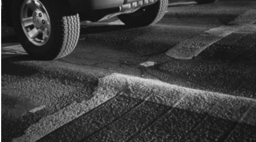
Figure 2-2: Severe rutting along the surface of a pavement (Paser Manual, 2002)
