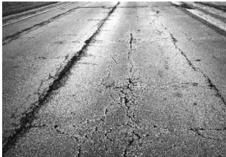
Figure 2-3: Longitudinal cracks (PASER Manual, 2002)
