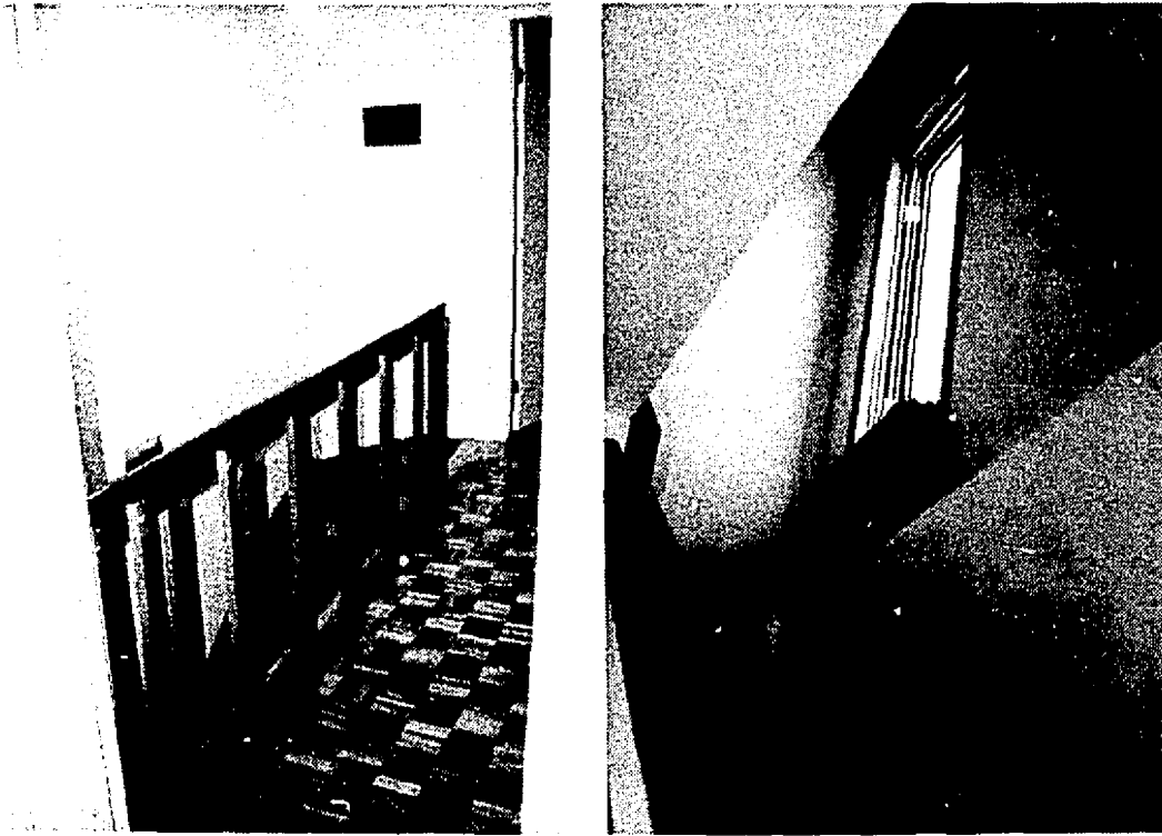
Fig. 4.32 The wall in the hallway was demolished and replaced by a wooden handrail (left). A window was added in the stairs area in order to make the room look more spacious, more attractive and to gain extra light (right).
